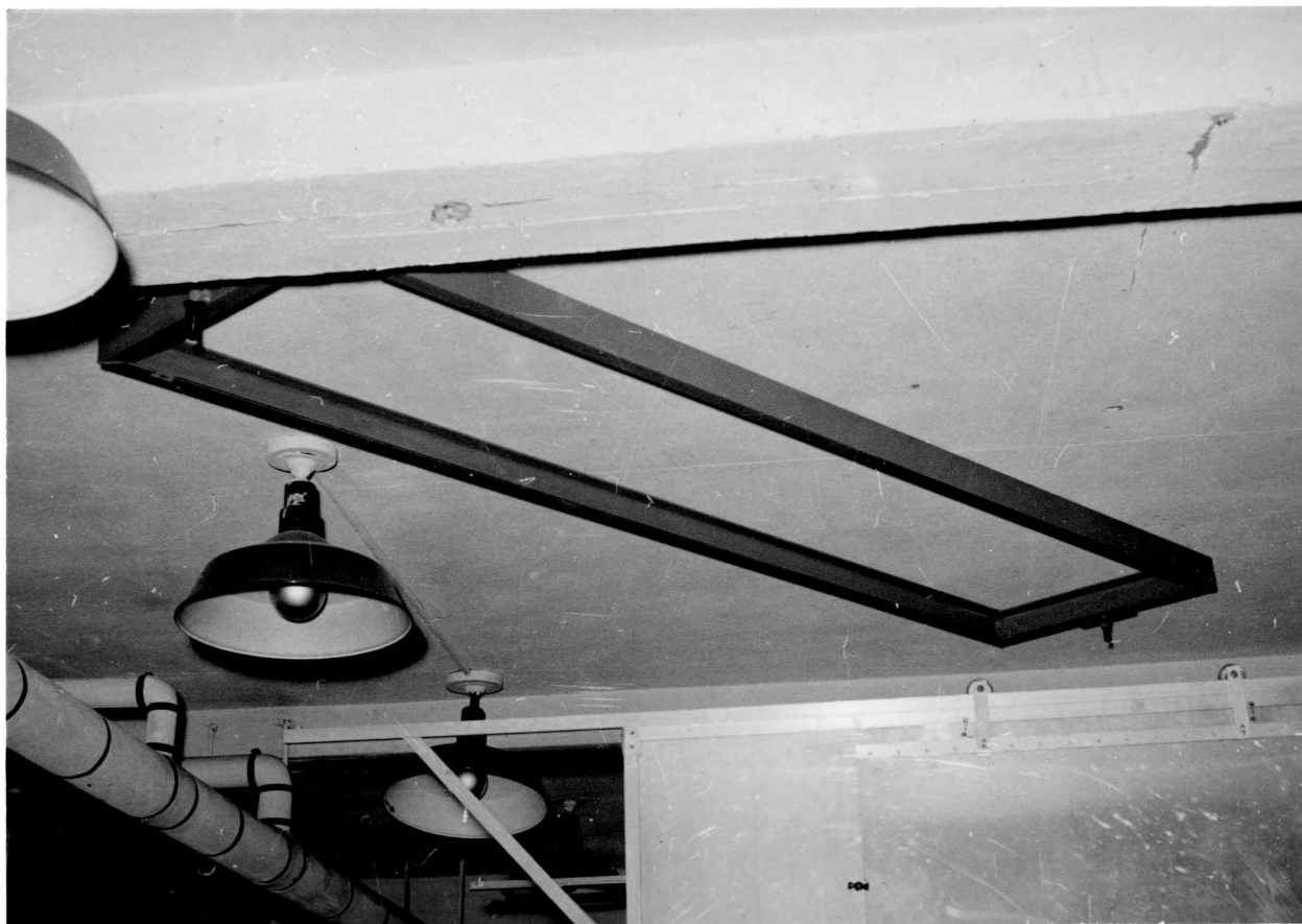
Figure 13. Mounting Track in Position Over Reactor.
