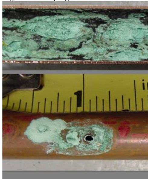
Fig. 2.4. Non-uniform (i.e., pitting) corrosion on copper tubing from a residence in a community with high water age.
