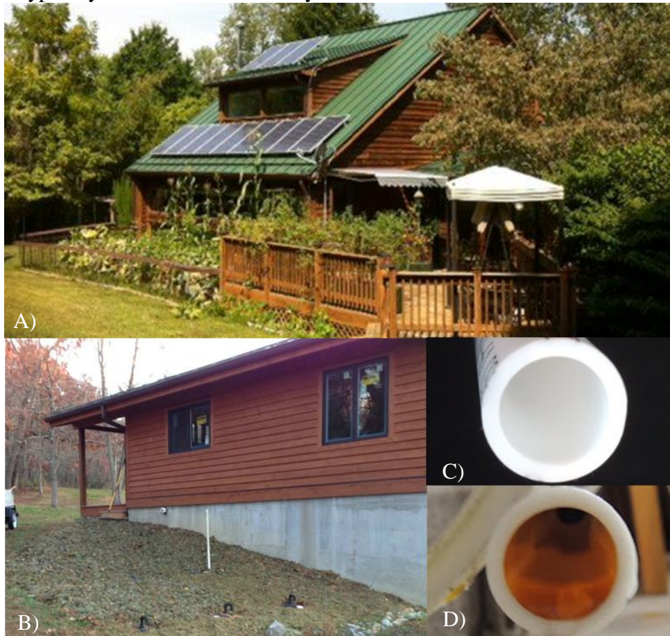
Fig. 2.5. Completely off-grid rainwater system
