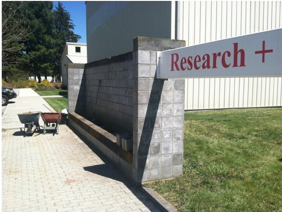
Figure 116: This is the front of the concrete block wall before constructing the Solar Lounge. The project serves as a test of many systems that might be included in the Solar Garage case study.
