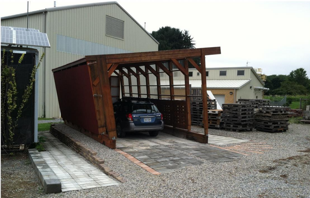
Figure 115: The current Solar Garage with my personal car testing clearance and for scale in Fall 2016 and the proof of the concept from another angle, testing the dropped floor design and concrete masonry unit distance and strength.. Due to the prolonged nature of the construction process with the Solar Garage and testing of the vegetated assembly system in the next case study: the Solar Lounge, vegetated assemblies have not yet been implemented on the structure.
