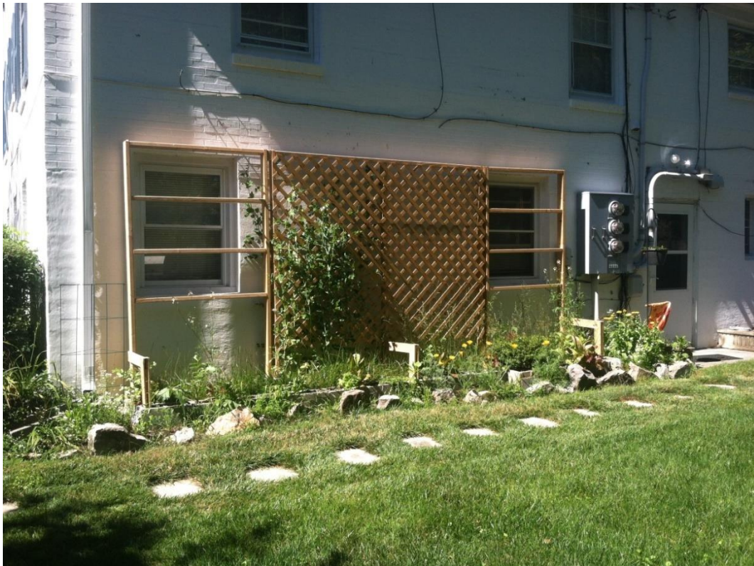
Figure 65-66: Turtletown before (above) and after (below). The materials were all laid out and over the course of a few hours were completely installed in our backyard. In July the selected vining peas had grown quite vigorously on the lattice and the mixed wildflowers began to bloom starting with yellows, changing to whites later on.
