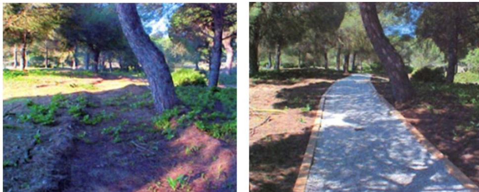
Figure 134: The before and after of the same area of the walking trail in Rota, Spain. This was the first time a project was constructed at full scale in a natural setting. The project had a large amount of help for a local Battalion of SeaBees (combat engineers for the Navy) who had heard about the free lunch offered.
