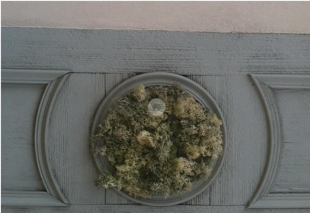
Figure 150: Not every vegetated assembly fills an entire wall. Some are humble such as this doorway insert of moss in Basel, Switzerland.
