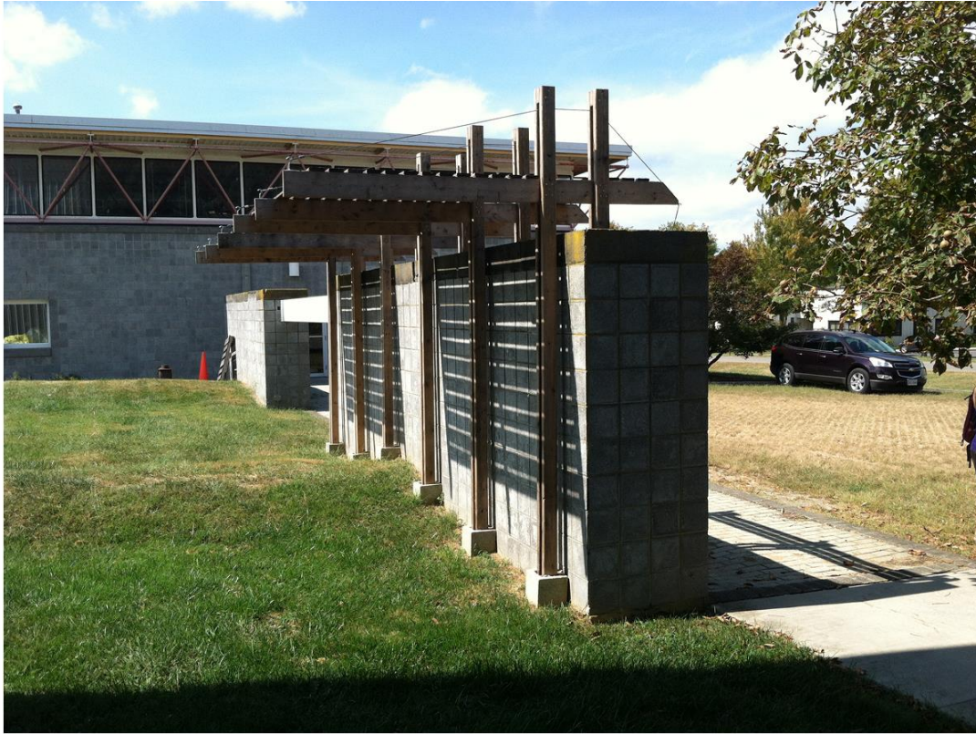
Figure 117: View towards the Research and Demonstration Facility after from constructing the Solar Lounge. The repeating frames of dimensional lumber provide a space for resting at RDF.
