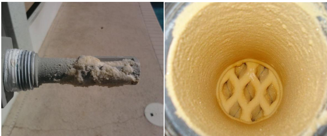
Figure 3-4. Calcite scale clogging chemical feed equipment (left) and pipes (right) at the school
