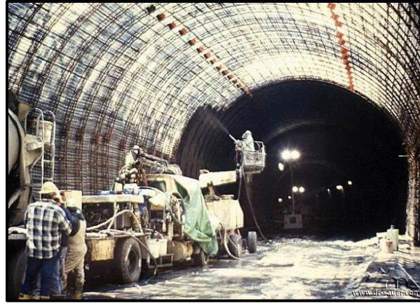
Figure 2-21. Shotcrete Application (Dr. Sauer Group, 2012)
