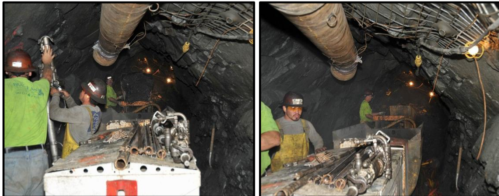
Figure 4-30. Traditional Drill and Blast Utility Tunneling (images courtesy of Howard County Public Utilities)
