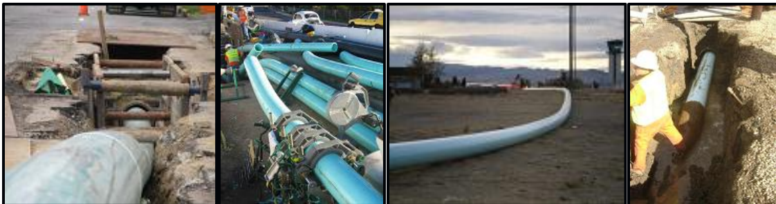
Figure 2-23. Insertion (left), Fusion (left-center), Lay-Down Area (right-center), Exit Pit (right) (Underground Solutions, Inc., 2011)
