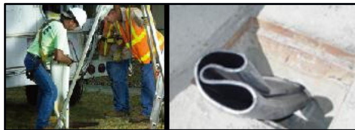
Figure 2-20. Thermoformed PVC Liner Insertion (left) (Miller Pipeline, 2012) and Deformed/Reformed Liner Exiting Pipeline (right) (HydroTech Inc., 2012)
