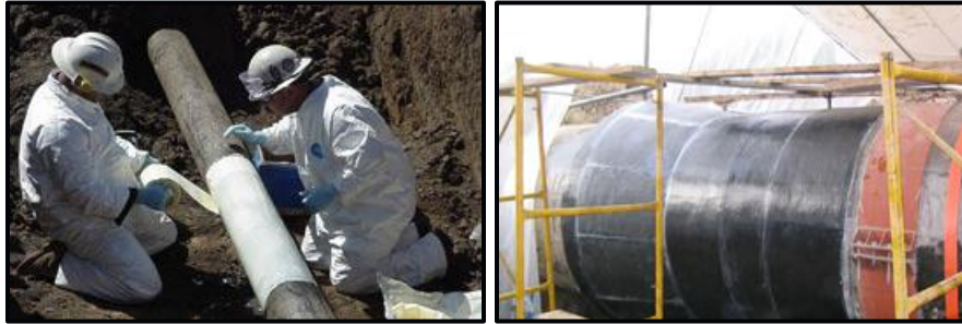
Figure 2-14. External Pipe Wrap Applications on Small Diameter (left) (EA Services, 2011) and large diameter (right) (Fyfe Co, LLC, 2009)
