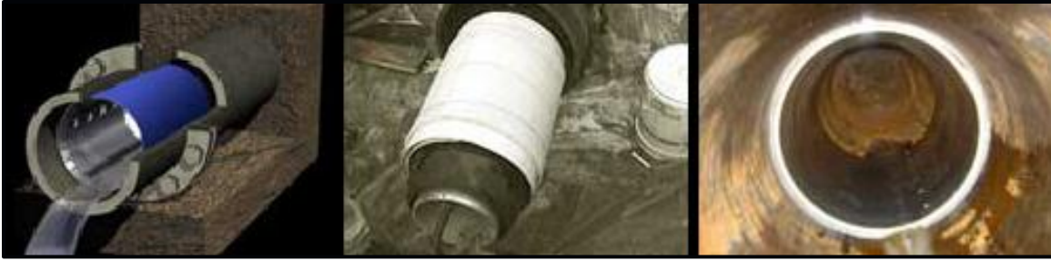
Figure 2-4. Mechanical Sleeve (left), Cured in Place Internal Sleeve (center), and Installed Sleeve (right) (Link-Pipe, 2010)
