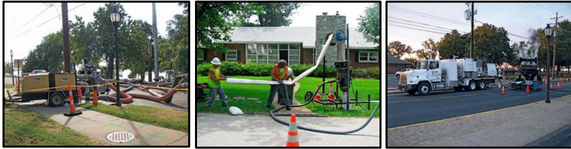
Figure 4-21. Temporary Bypass (left) and CIPP Installation in the City of Henderson (center and right) (images courtesy of the City of Henderson)
