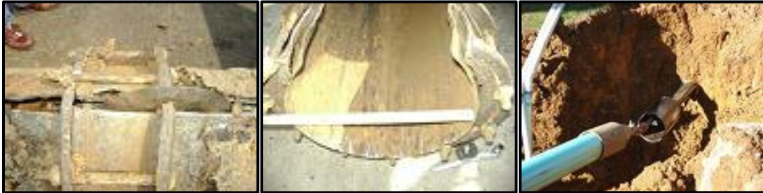
Figure 2-30. Cutter Head at Coupling (left), Expanded Steel Pipe (center), Bursting Head (right) (Underground Solutions, Inc., 2011)
