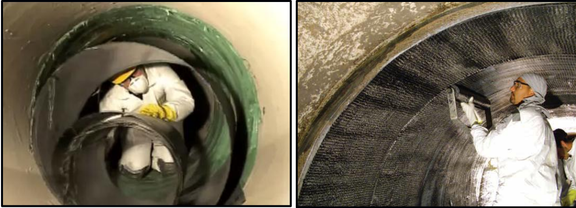
Figure 2-8. Fiber Reinforced Internal Pipe Wrap – Pre-Cured Laminate (left) (Pipe Medic, LLC, 2012) and Wet-Lay Up Applied (right) (Fyfe Co, LLC, 2009)
