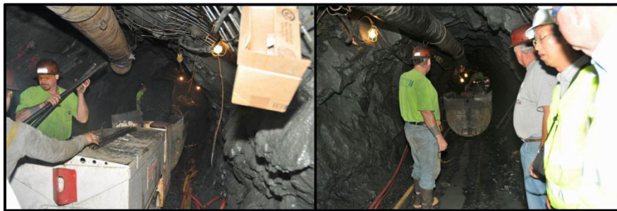
Figure 2-36. Back Dump Mucker to Remove Debris (left) and Dumping of Spoil into Muck Car (right) (Steiner, Sewer Interceptor Installation Using Traditional Drill and Blast Tunneling Techniques in Howard County, MD, 2012)
