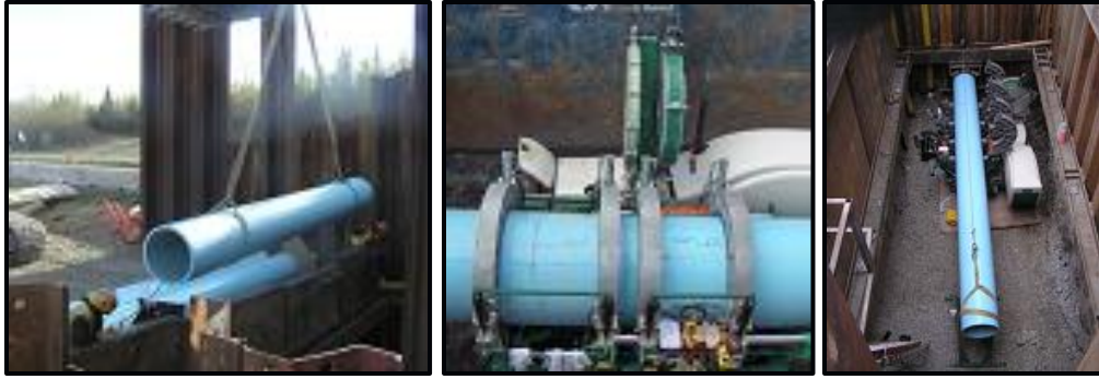
Figure 2-22. Loading of Pipe Segment into Fusion Pit (left), Fusion (center), and Insertion (right) (Underground Solutions, Inc., 2011)
