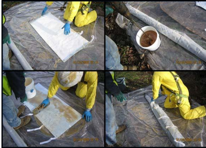
Figure 2-10. CIPP Short Liner Material (top left), Mixing of Resins A and B (top right), Resin Application (bottom left), Liner Secured to Carrier Tube (bottom right) (Steiner, 2012)
