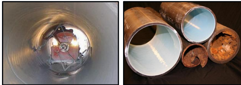
Figure 2-15. Cementitious Coating (left) (Cement Lining Corporation International, 2008) and Epoxy Coating (right) (Craftsman Pipe Lining, Inc., 2012)
