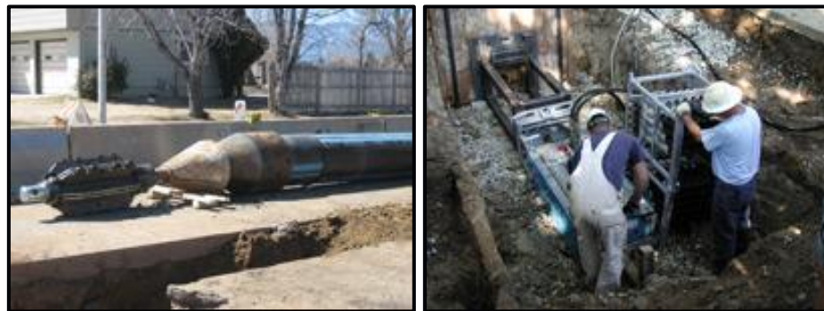
Figure 2-33. Static Pipe Bursting Head (left) and Bursting Machine (right) (TT Technologies, Inc., 2012)
