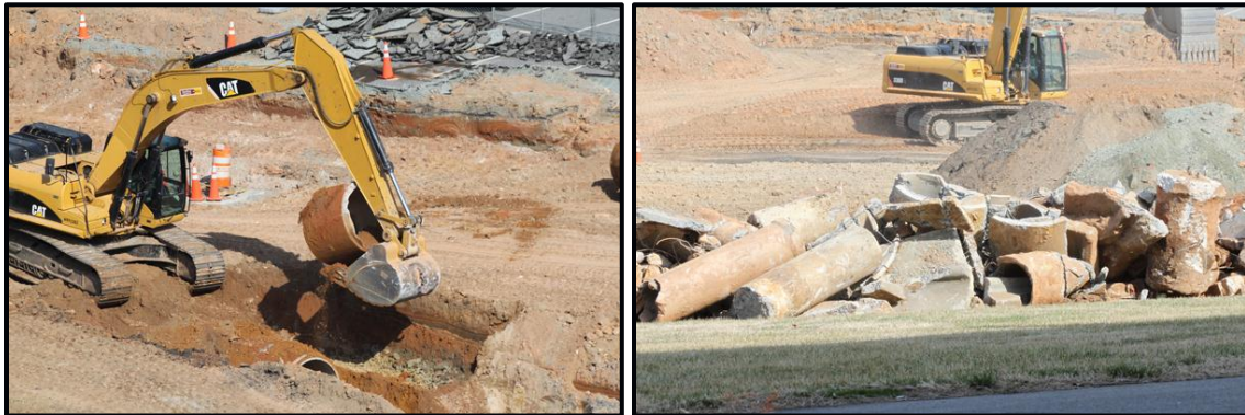
Figure 2-35. Exhume and Replace Pipe Removal (Wake Forest, 2011)
