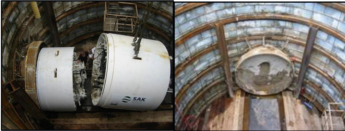
Figure 2-37. Microtunneling Machine (left) and Access Shaft (right) (SAK Construction, 2012)
