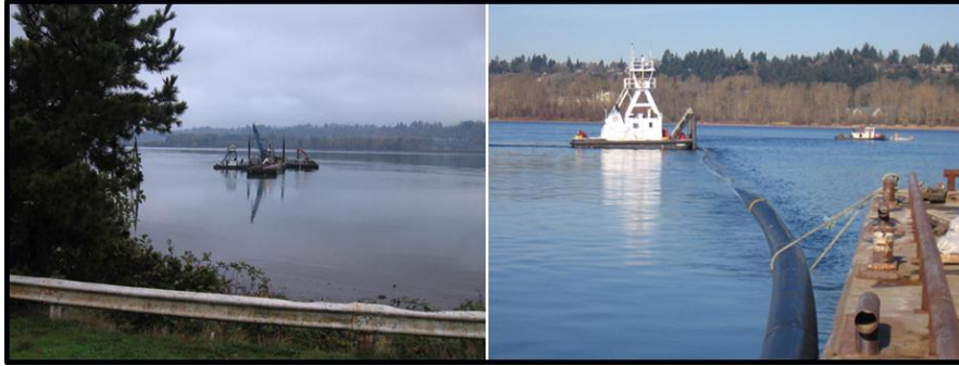
Figure 4-31. Barge on Columbia River (left) and Pull-In of 30" HDPE Pipe at Columbia River Outfall (right) (Kinnan Engineering, Inc., 2009)
