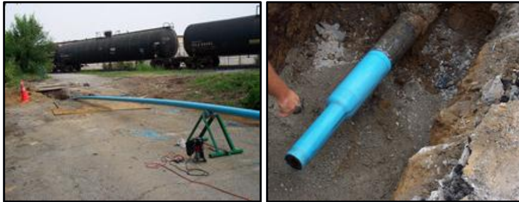
Figure 2-25. Expand-in-Place PVC Entering Host Pipe (left) and After Expansion (right) (Underground Solutions, 2012)
