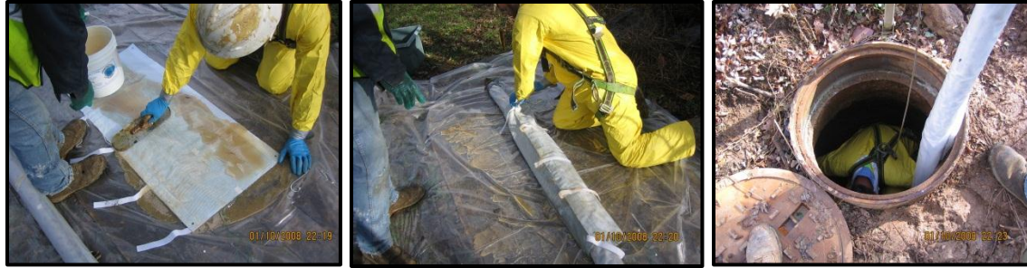
Figure 4-16. Resin Application (left), Wrapping of Liner on Inflatable Device (center), and Insertion of Liner into Manhole (right) (images courtesy of the Metropolitan Sewerage District of Buncombe County, NC)
