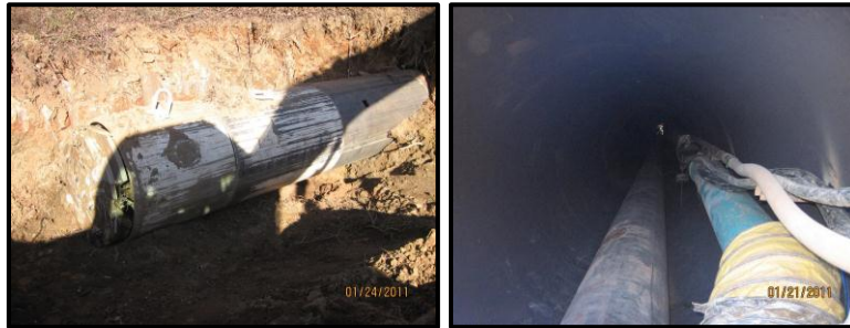
Figure 4-29. Auger Boring Machine at Receiving Pit and Installation of Carrier Pipe in Encasement Pipe (images courtesy of the Metropolitan Sewerage District of Buncombe County, NC)
