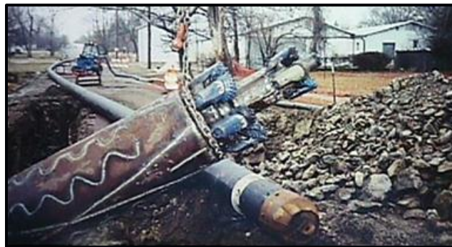
Figure 2-34. Reaming Head Recommended for Use with VCP (Nowak Pipe Reaming, Inc., 2011)
