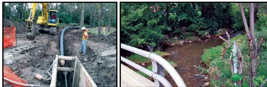
Figure 4-33. HDD Crossing of Stream in Villa Park, IL
