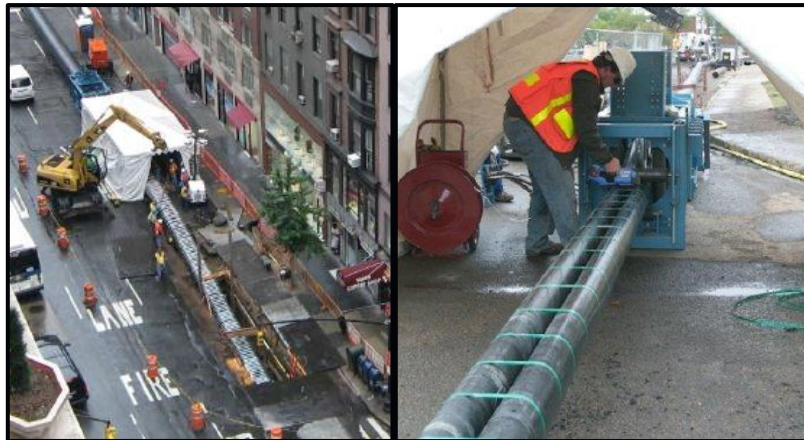
Figure 2-24. On-Site Deformation of Deformed HDPE Pipe Liner Pull-In (left) and Close-Up of Deforming Machine (right) (Insituform Technologies, Inc., 2012)
