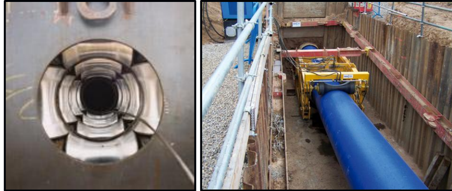
Figure 2-26. Mechanical Radial Reduction by Compression (left) (Insituform Technologies, Inc., 2012) and Tension (right) (Swagelining, 2011)
