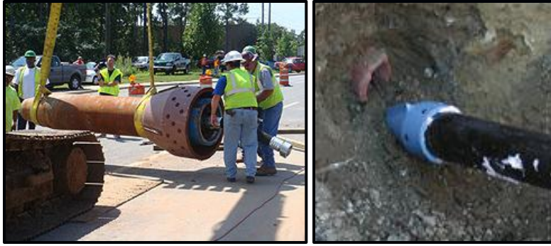
Figure 2-31. Pneumatic Bursting Head (TT Technologies, Inc., 2012)
