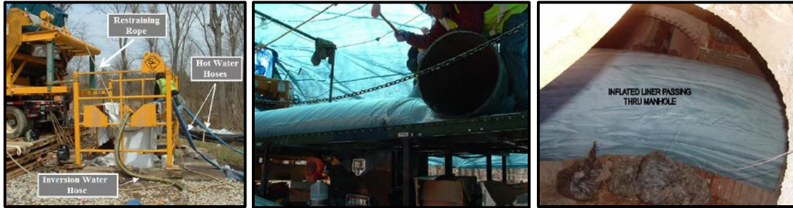
Figure 4-22. Inversion Equipment Setup, Dispersion of Resin after Impregnation, and Inflated Liner Passing through Manhole (images courtesy of Baltimore County)
