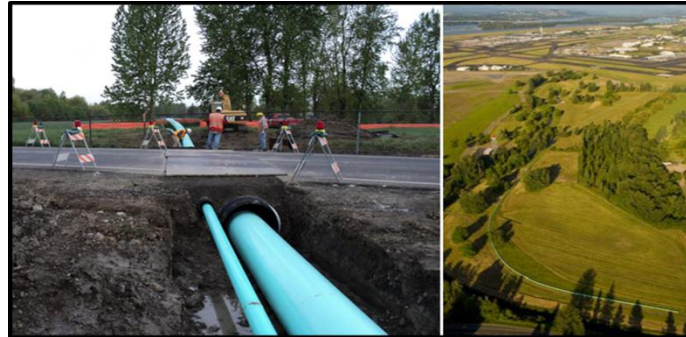
Figure 4-32. Duel Pipe String Passing Through Culverts (left) (Kinnan Engineering, Inc., 2010), Pipe Lay-Down Area (right) (Jack R. Ostlund, 2011)
