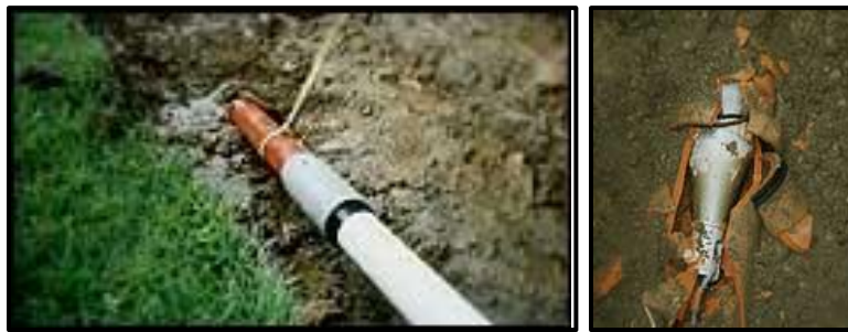
Figure 4-27. Launch Pit and Bursting Head in Benton, AR Pipe Bursting Project (images courtesy of the City of Benton) (TT Technologies, Inc., 2011)
