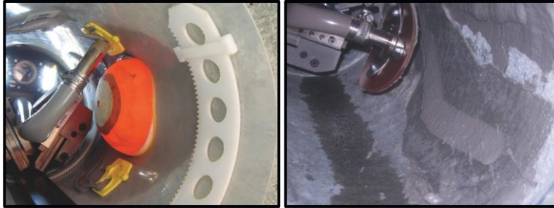
Figure 2-11. Resin Injection (Heenan, 2010)
