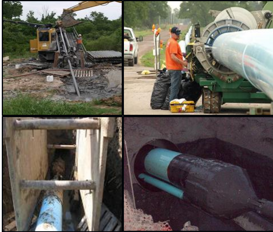
Figure 2-38. Drilling Rods and Rig (top left), Pipe Fusion (top right), Pipe Pull-In (bottom left), Exit Pit (bottom right) (Underground Solutions, Inc., 2011)
