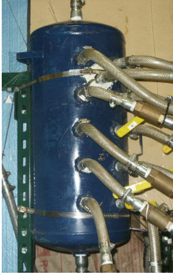
Figure 3-23 “Octopus” microcircuit coolant flow plenum. Air enters through the tubing above and below, and exits through the nine valved exit hoses.
