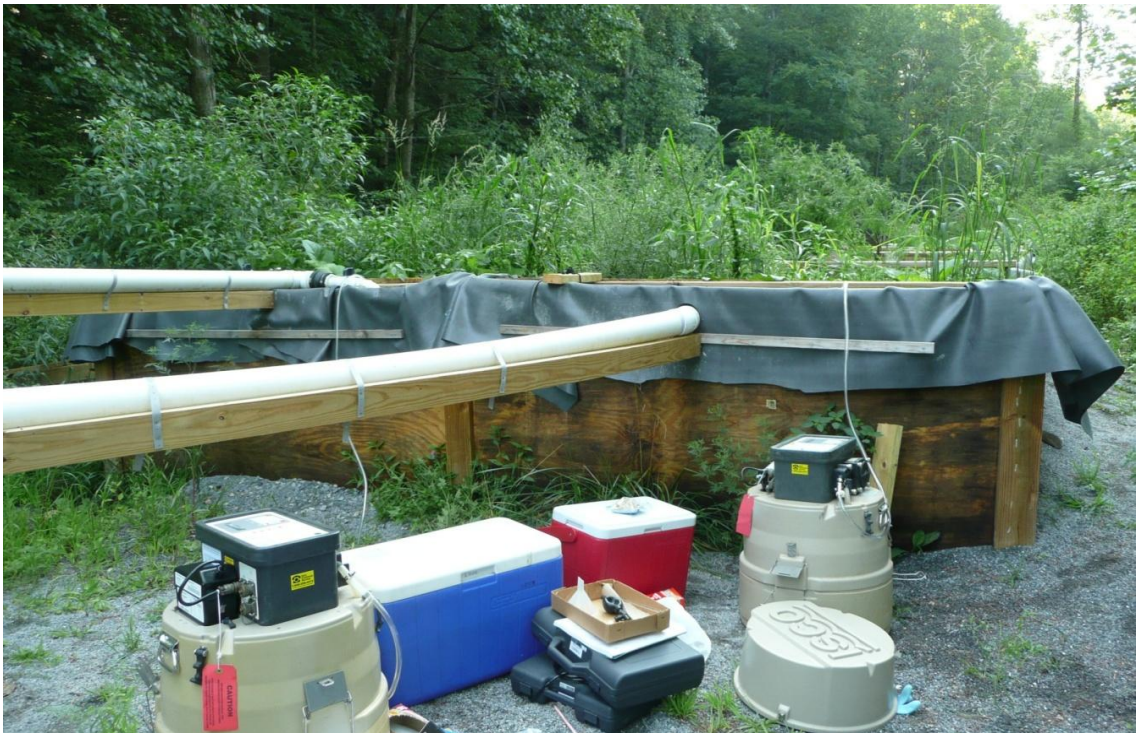
Image 4: Front view of constructed wetlands
