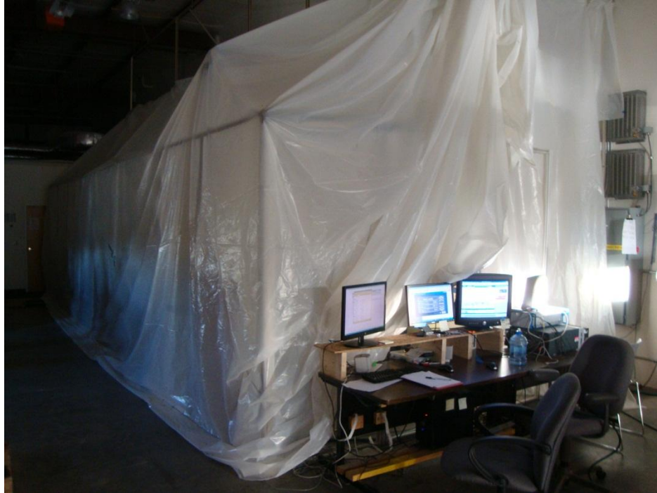
Figure 5-4. The plastic sheeting surrounding the enclosure.
