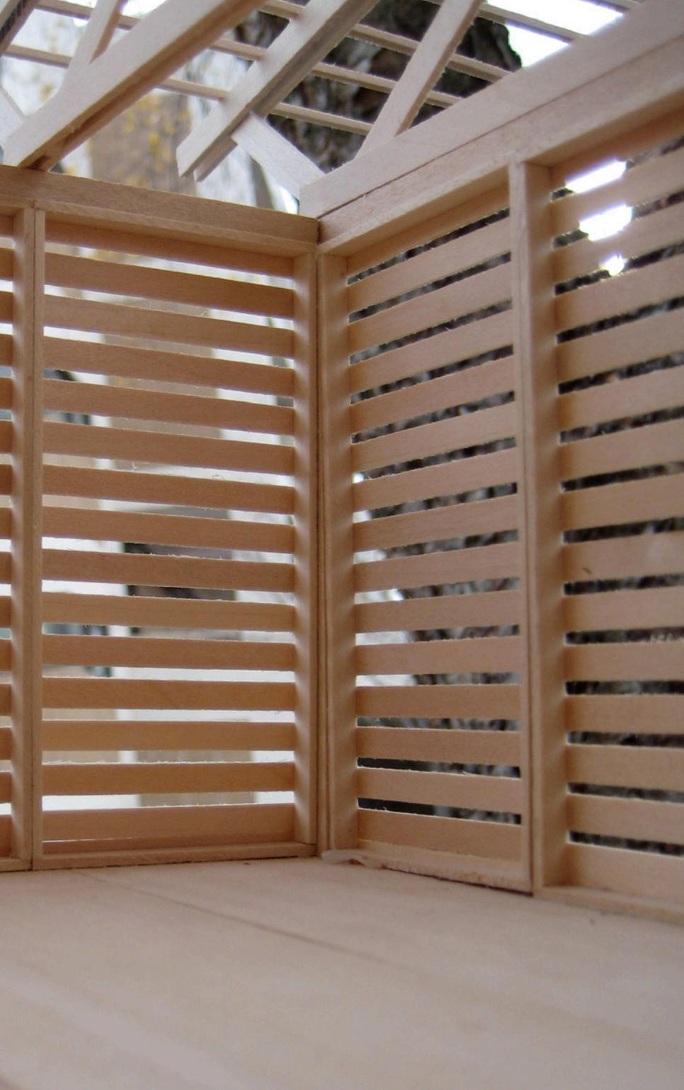
dry air from all sides of the building. Often the Corn Cribs foundation is inboard of the roof perimeter, which allows the side to slope outward. The sloping sides serve to increase the surface area of ventilation as well as protect the corn near the bottom from rooftop rainwater run off.
