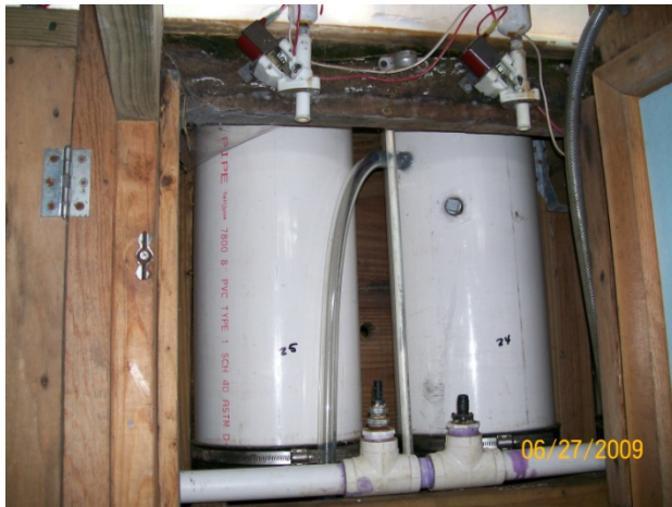
Figure 3. Close-up of PVC pipe columns. Notice the black rubber covering on the bottom of the pipes
