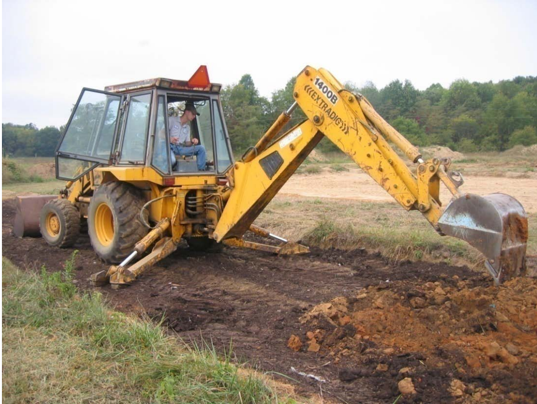
Figure 24. Excavating compacted soil and mixing compost into profile.
