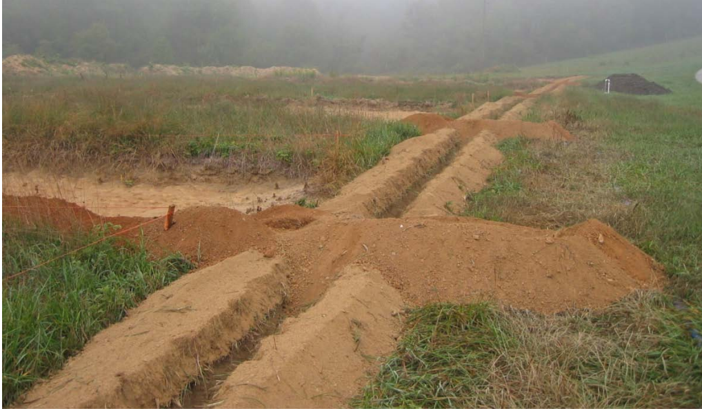
Figure 4. Drainage ditch installation at the western edge of each undisturbed plot after pre-treatment due to the raised surface of the undisturbed topsoil.
