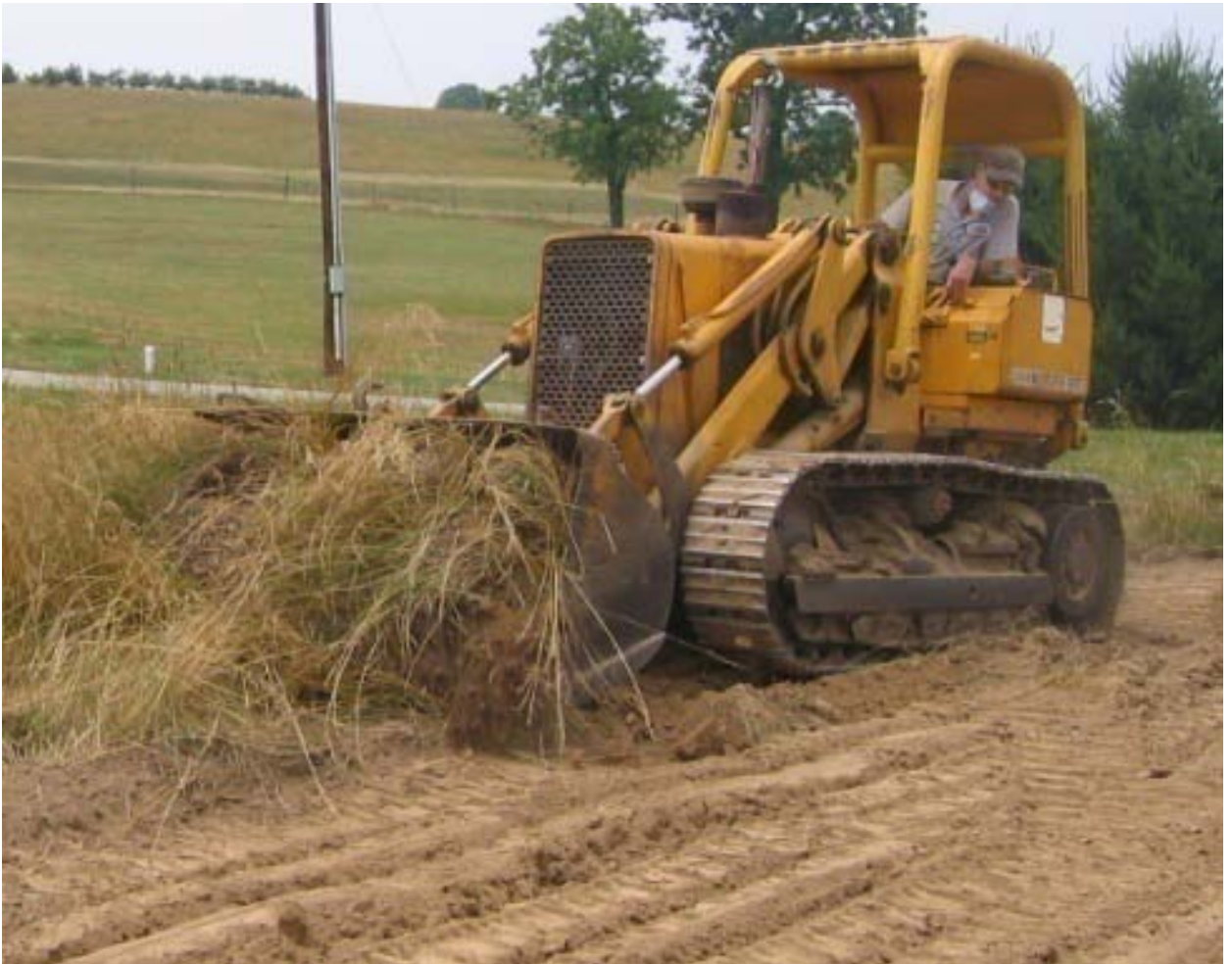
Figure 10. Scraping initial layer of topsoil with vegetation June 19, 2007.
