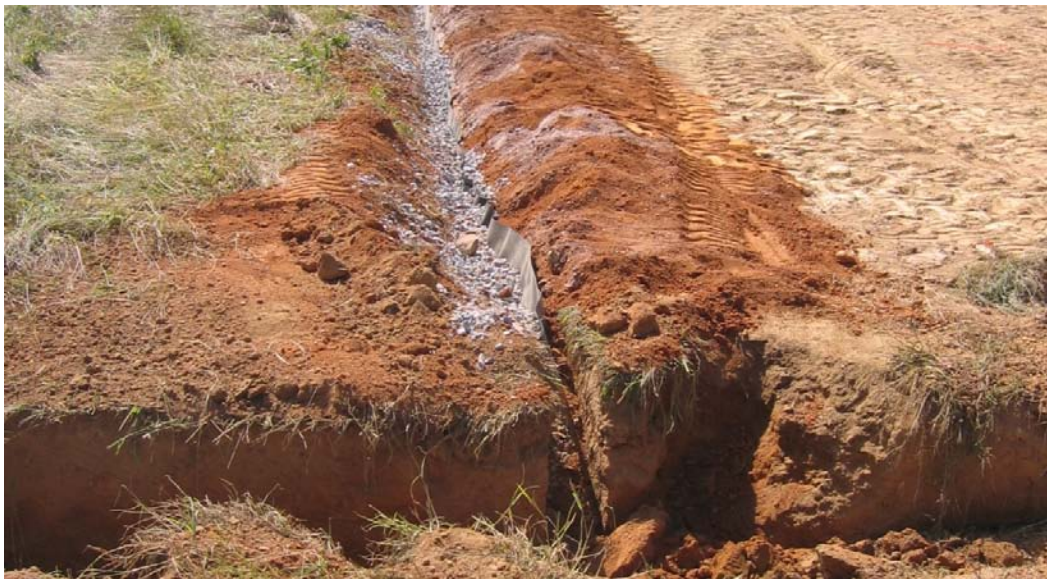
Figure 5. Drainage ditch installation to aid in drainage created at the western edge of each undisturbed plot after pre-treatment due to the raised surface of the undisturbed topsoil.
