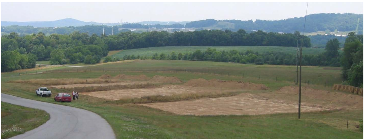
Figure 12. After scraping and stockpiling topsoil June 28, 2007.
