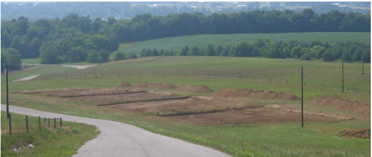
Figure 16. After compaction on July 5, 2007.
