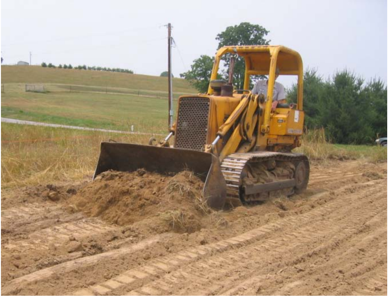
Figure 11. Scraping 25-30 cm topsoil June 19, 2007 driven by Chad Keith.
