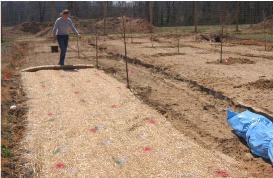
Figure 27. Placement of erosion control mats.
