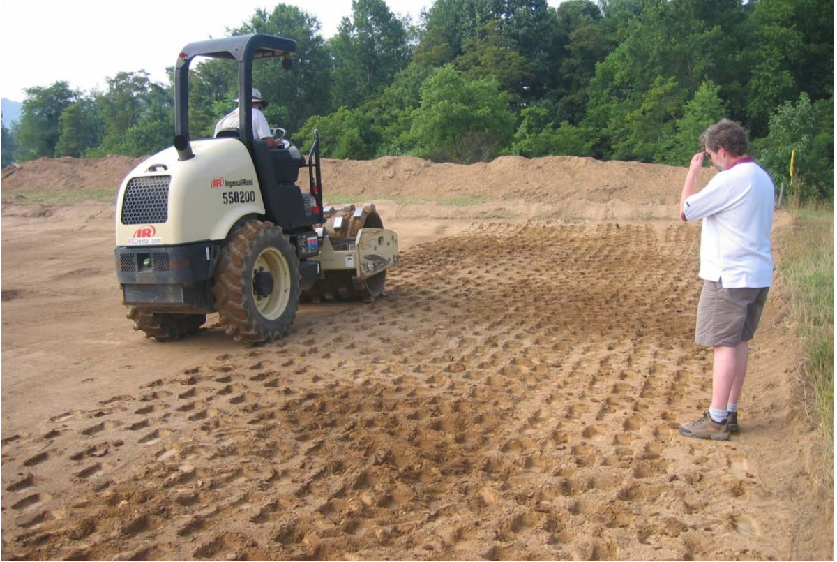
Figure 15. Dr. Lee Daniels confirms soil moisture for compaction on July 5, 2007.
