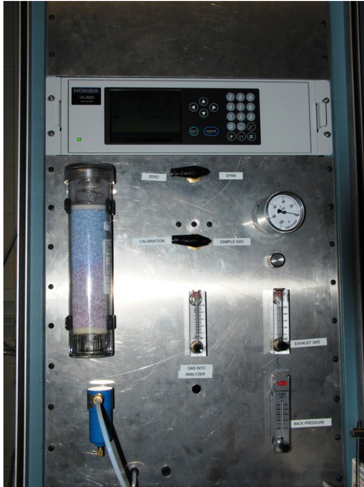
Figure 17. Control panel of the cone calorimeter.
