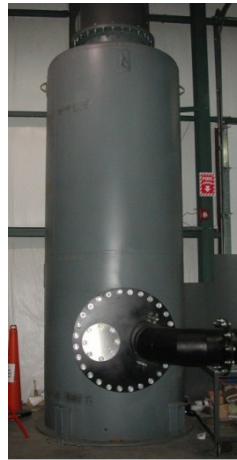
Figure 2–6: The exhaust section of the facility connects to the silencer which muffles noise created by the exiting flow
