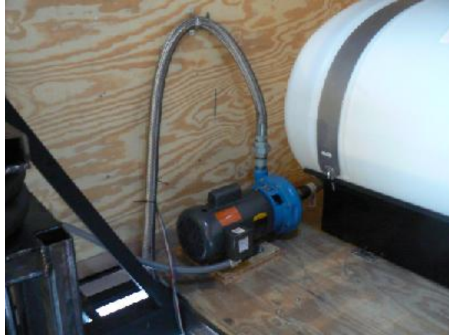
Figure 24. Goulds Pump Mounted in the Front of TTT. [Photo by author 2009]
