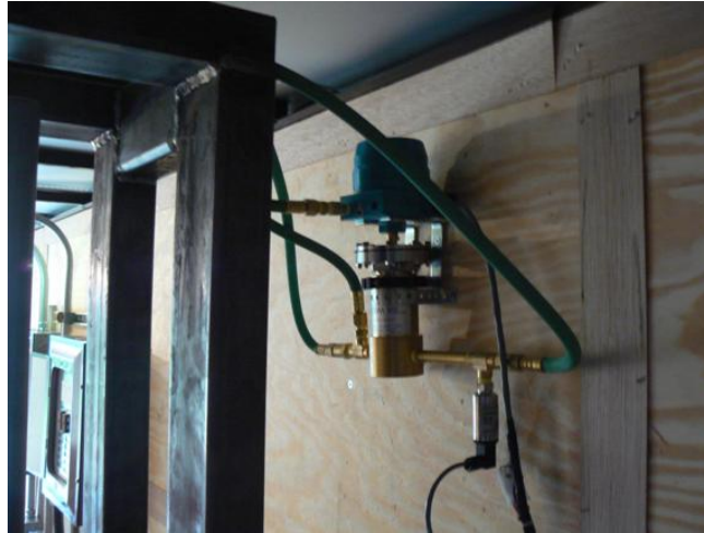
Figure 17. Pneumatic Regulator Mounted in TTT. [Photo by author 2009]
