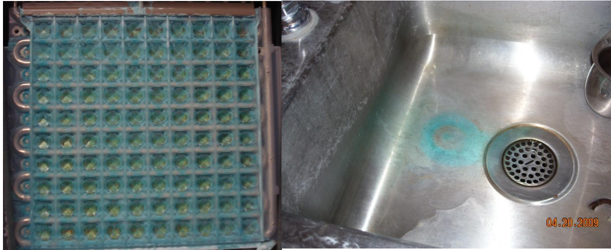
Figure 1-1. Pictures of blue ice cubes from Miami Public School and blue staining in sink.
