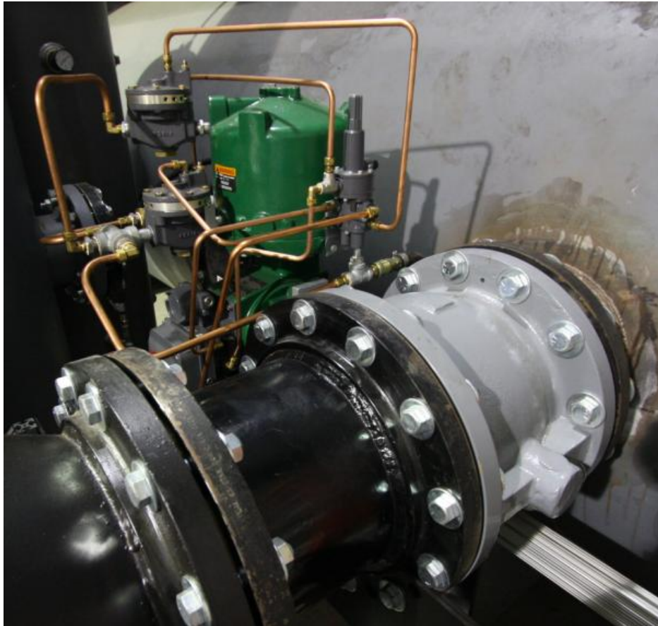
Figure 2.2. Fisher 12" Vee-Ball Control Valve and inlet pipe to supersonic wind tunnel wide angle diffuser. The valve components and copper tubing attached to the body are the volume boosters, and safety trip valve.
