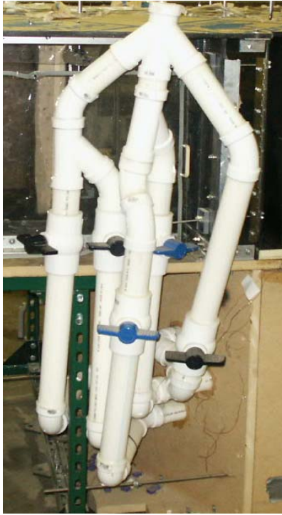
Figure 3.22 Picture of five PVC valves for each of the plenums fed by one compressed air line.
