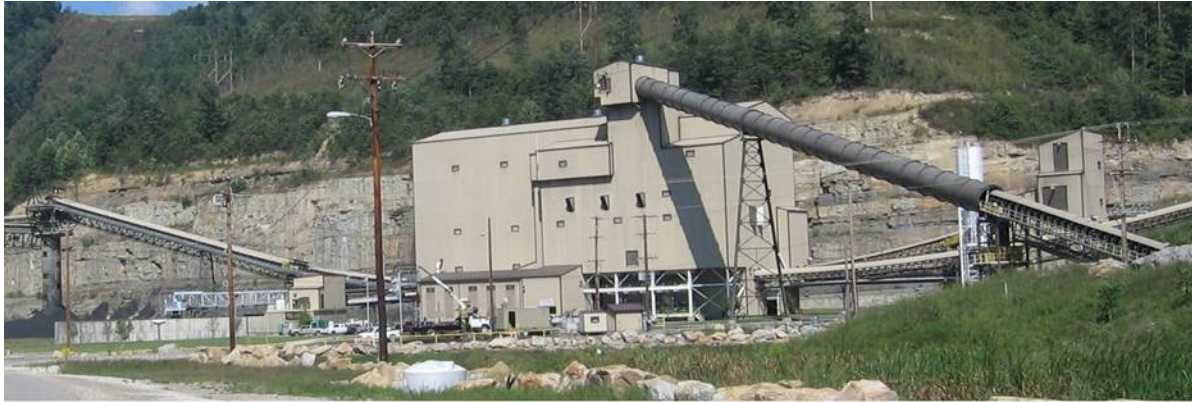
Figure 4.4 Cardinal Preparation Plant, WV.
