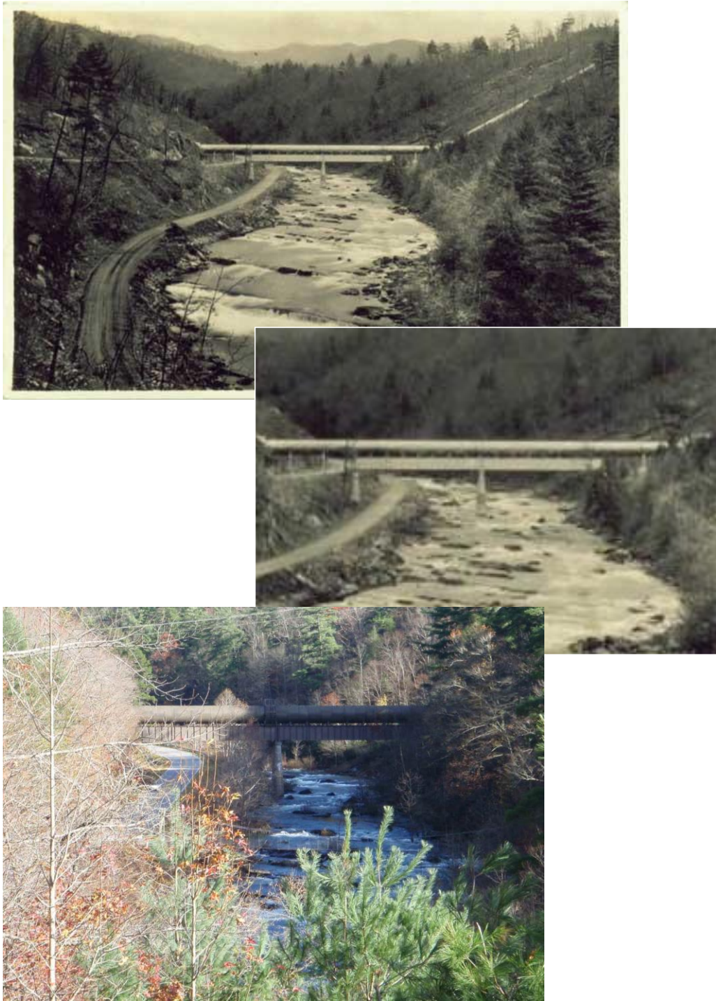
Figure 6.12 Postcard from the 1930's of the lower penstock crossing on the Cheoah River soon after the dam completion (1927) (top) (source: http://www.tailofthedragon.com ). Serial photos of the channel under the penstock crossing in 1930's (middle) and in 2009 (bottom).
