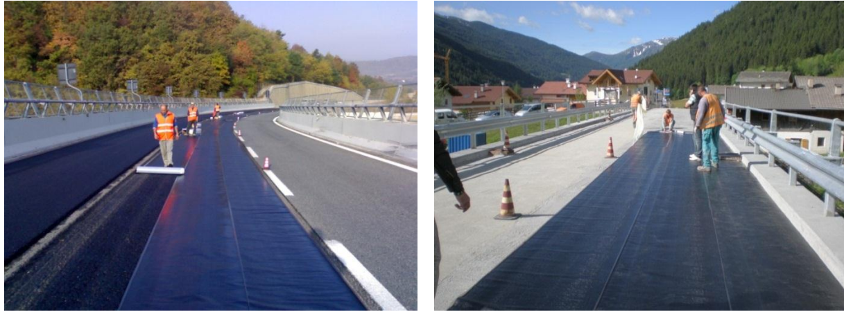
Figure 2.2: a) Full scale test area, highway; b) Full scale test area, local mountain road.
