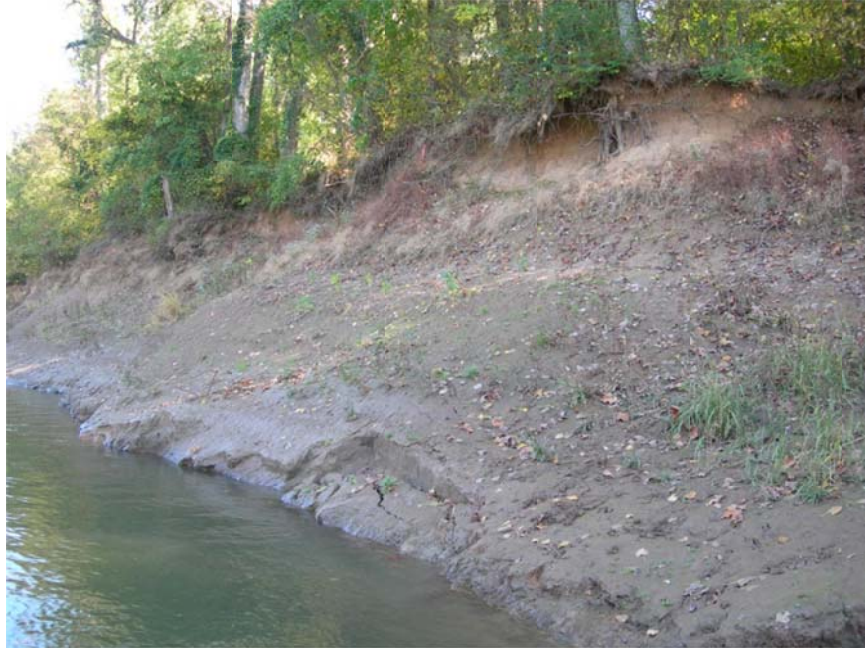
Figure 2 A segment of the riverbank along the Lower Roanoke River in North Carolina that has undergone extensive erosion and bank instability. Soil samples from this site were used in the present study.
