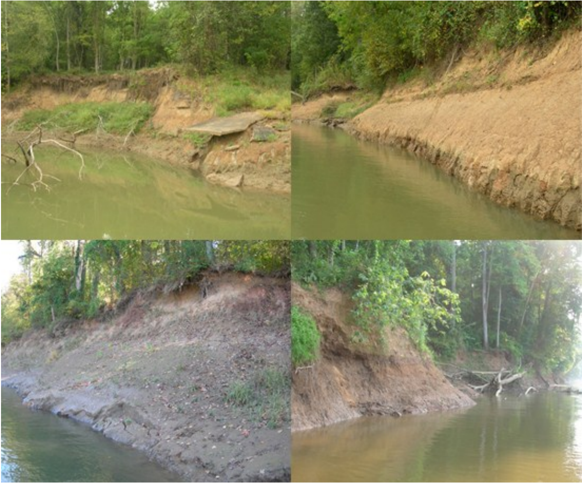
Figure 2 Severe erosion and bank failures near study sites in the lower Roanoke River, NC.
