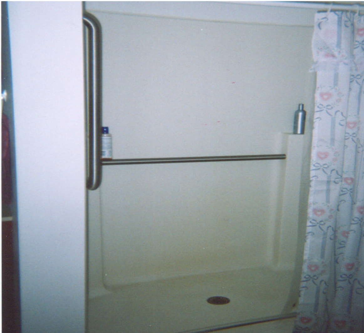
Figure 19 - Plan A Shower Grab Bars and Two Shower Rods
