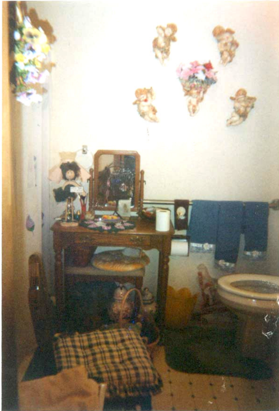
Figure 33 – Plan B Bathroom - No Clear Approach to Toilet
