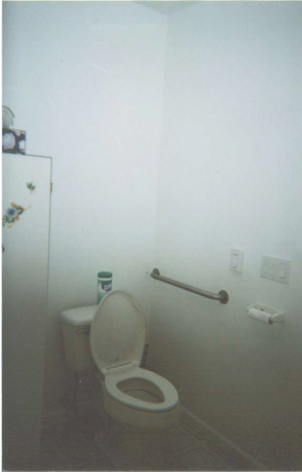
Figure 21 - Plan A Toilet Clear Space and Grab Bars
