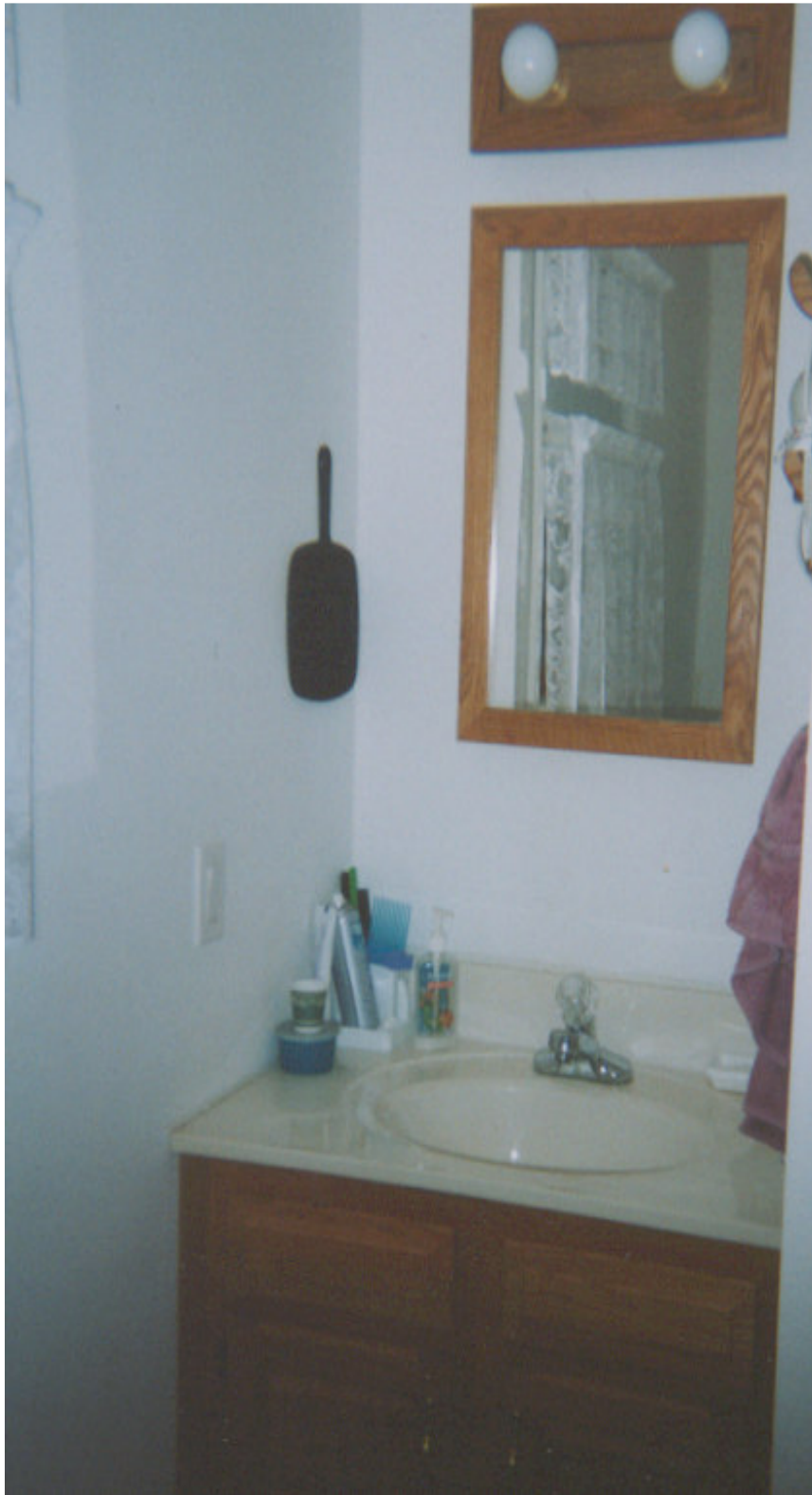
Figure 20- Plan A Bathroom Vanity No Clear Knee Space
