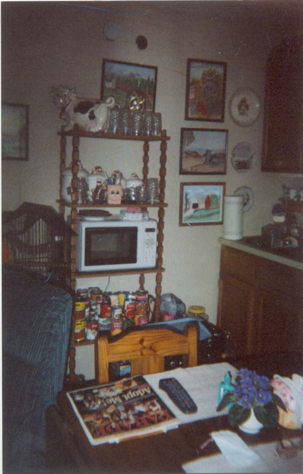
Figure 26 – No Clear Circulation Space in Task area of Kitchen
