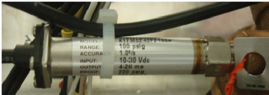
Figure 5.13. Image of the pressure transmitter.
