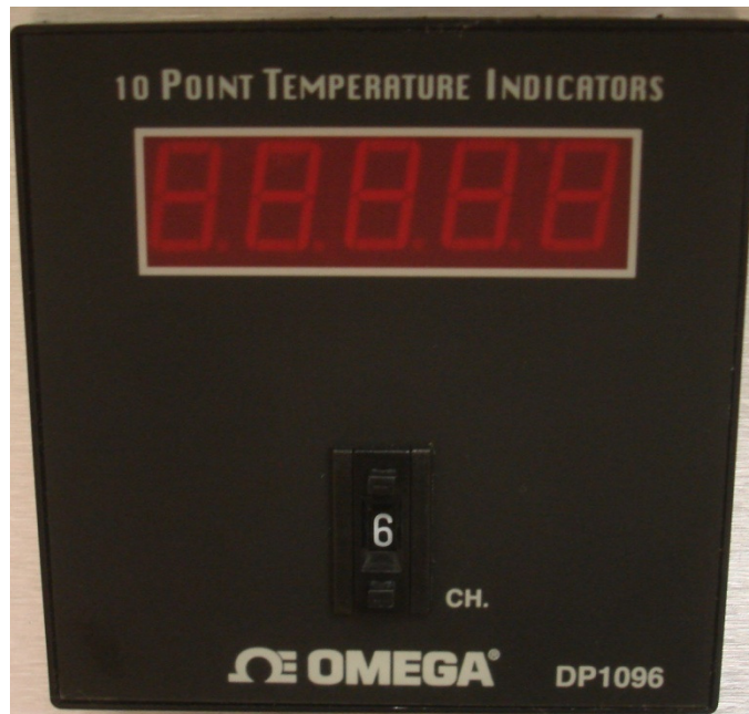
Figure 5.15. Image of the ten point temperature indicator.
