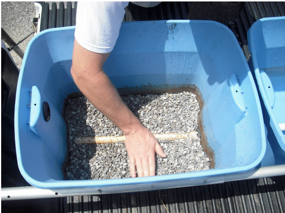
Incomplete bottom gravel layer showing outlet structure
