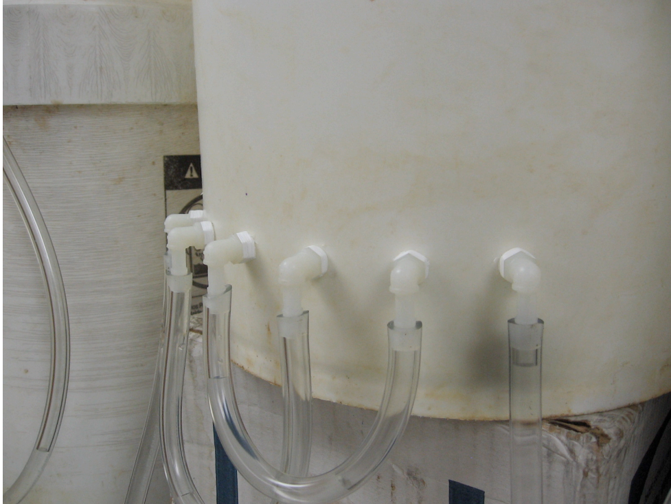
Completed fittings on the constant head tank
