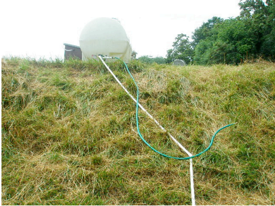
Location of the head tank atop the earthen embankment of the pond
