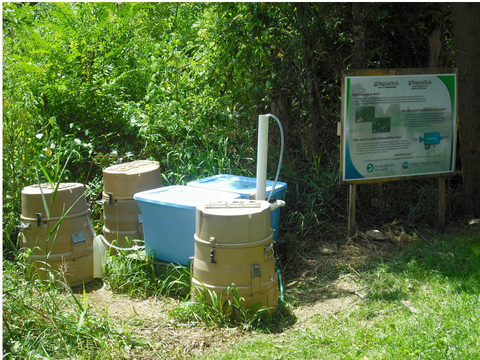
Filtration setup at the retention pond with two experimental cells, inlet structure, and automated samplers
