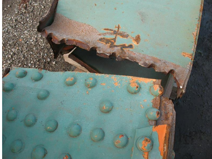
Figure 4-2. Wreckage of member U10U11 on the East side of the main truss. NTSB (2009). Collapse of I-35W Highway Bridge, Minneapolis, Minnesota, August 1, 2007. National Transportation Safety Board. Used under fair use, 2015.
