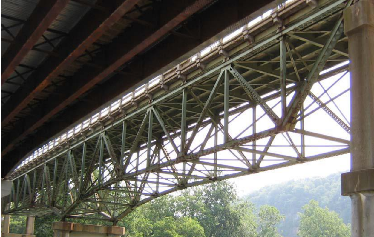
Figure 7-66. The main span truss structure of the New River Bridge. Hickey, L. J., et al. (2009). Live Load Test and Failure Analysis for the Steel Deck Truss Bridge Over the New River in Virginia. Report No.: FHWA/VTRC 09-CR8. Virginia Transportation Research Council. Charlottesville, VA. Used under fair use, 2015.
