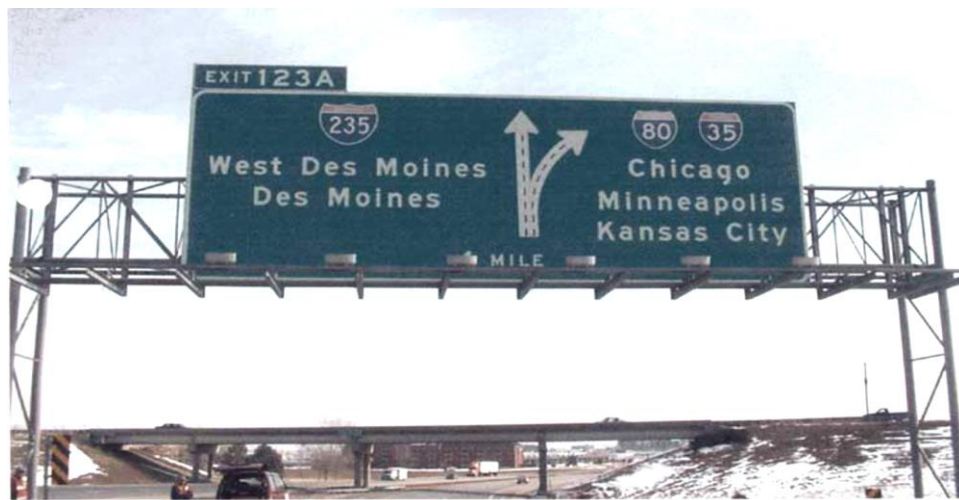
Figure 2-5. Close-up view of Interstate 80 Sign Truss. Wipf, T. J. and B. M. Phares (2002). Evaluation of Interstate 80 Sign Truss. The Iowa Department of Transportation. The Bridge Engineering Center at the Center for Transportation Research and Education-Iowa State University. Used under fair use, 2015.
