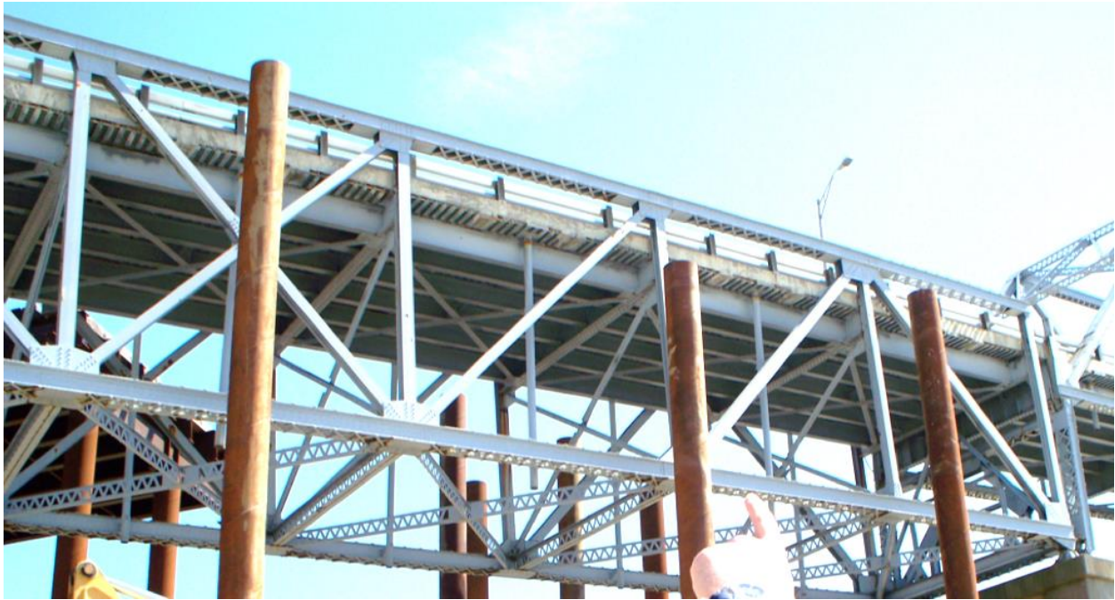
Figure 7-7. A side view of truss members and connections ( http://www.miltonmadisonbridge.com/gallery/ )
