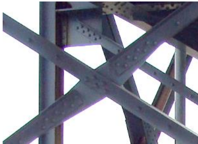
Figure 7-8. A close-up view of the connection details for a typical X-brace assembly. Diggelmann, L. M., et al. (2012). Evaluation of Member and Load-Path Redundancy on the US-421 Bridge over the Ohio River. Purdue University. Used under fair use, 2015.
