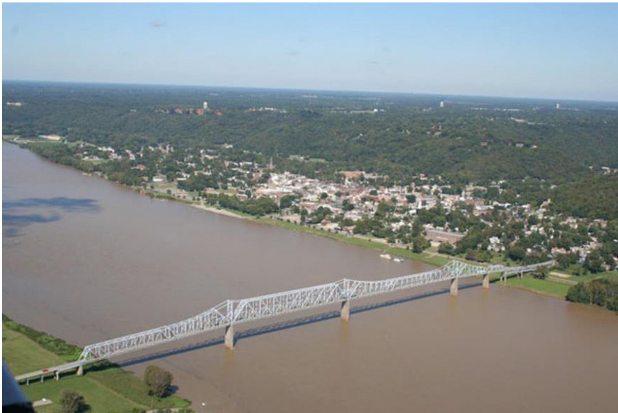
Figure 7-1. An aerial view of Milton-Madison Bridge ( http://www.miltonmadisonbridge.com/the-project/ )
