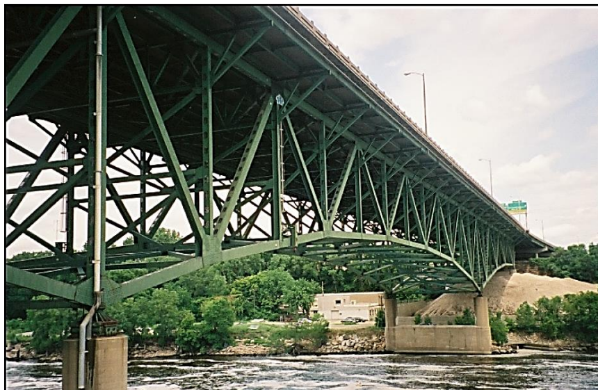
Figure 3-1. A side view of the I-35W Bridge. NTSB (2009). Collapse of I-35W Highway Bridge, Minneapolis, Minnesota, August 1, 2007. National Transportation Safety Board. Used under fair use, 2015.
