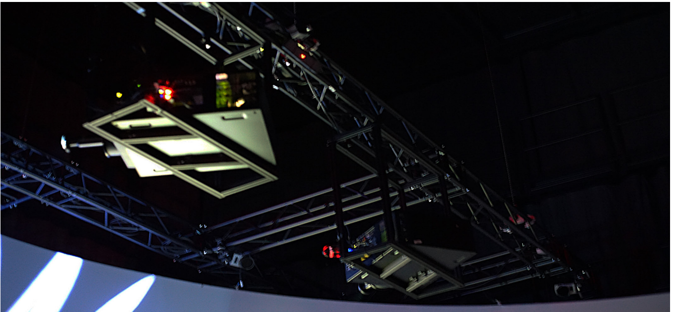
Figure 9.1: Dual projector setup attached to scaffolding above the Cyclorama.
