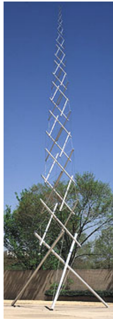
Figure 1.1: The Needle Tower at Hirshhorn Museum and Sculpture Garden in Washington D.C., created by Kenneth Snelson in 1968 using aluminum and stainless steel. The structure itself stands at 60 feet in height.[1]
