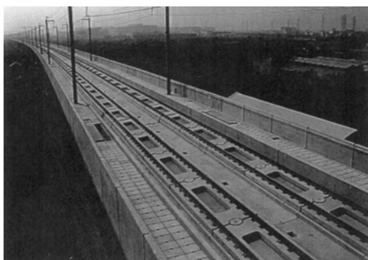
Figure 6. 3 J-Slab Rail Bed (public domain)
