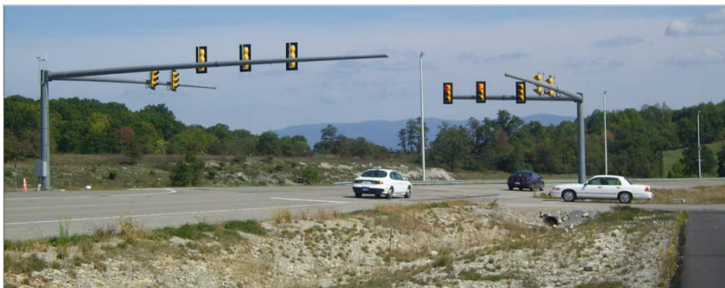
Figure 9: Signalized Intersection at Testing Site
