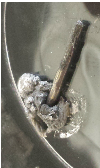
(a) Aluminum Wire Beginning to Corrode
