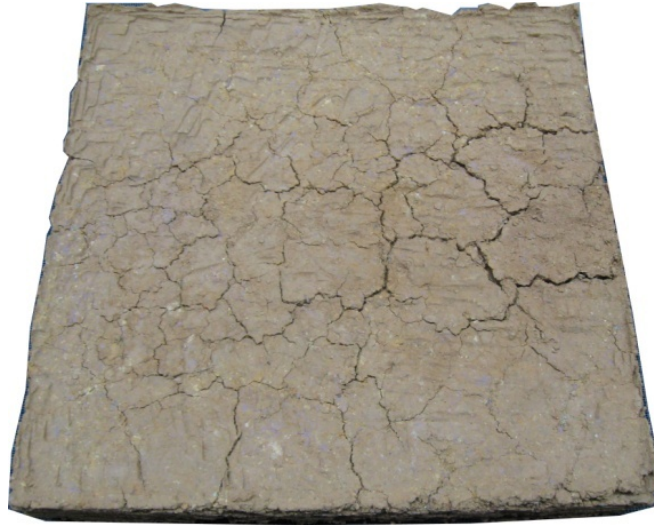
Figure 5.6: Image showing intensity of cracks on the surface of Panel-4 Earth + Clay + Elmer's glue
