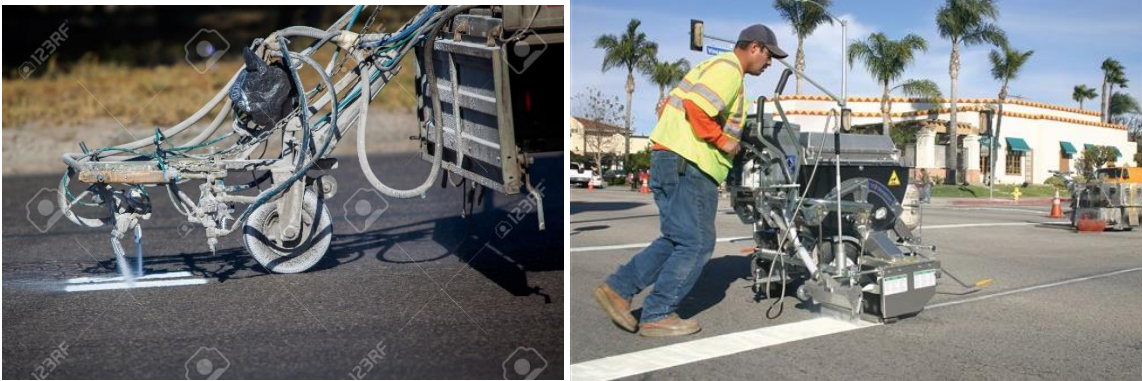
Figure 1.1 Road Working Zone for Paint Work 1
