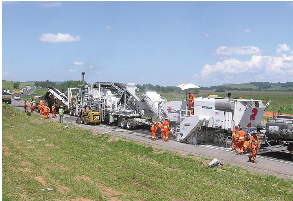
Figure 14: Cold Recycling Equipment on site
