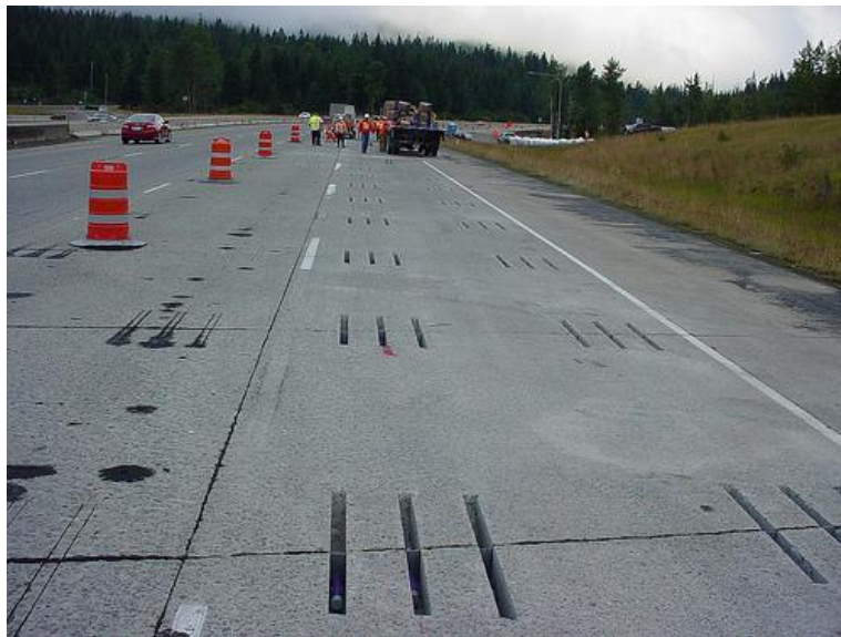
Figure 6: Slots along each wheel path
