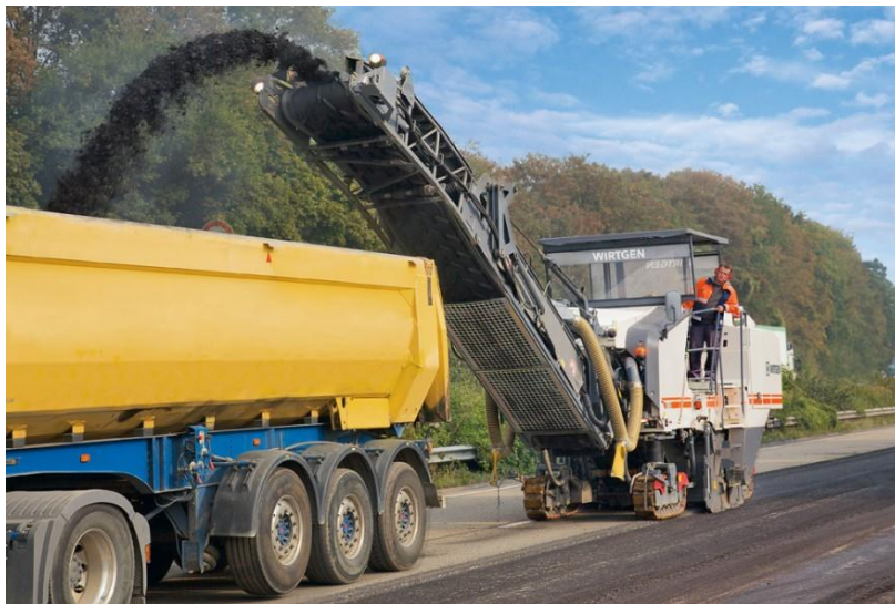
Figure 13: Cold Milling of Asphalt pavement
