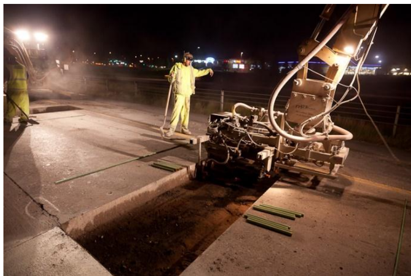
Figure 9: Removing slab for replacement
