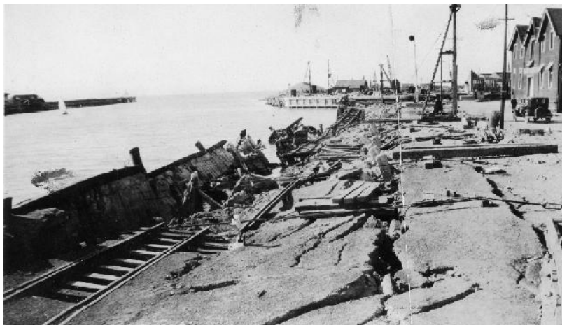
Figure B.1: Lateral spreading of the wharf in Ahuriri ( from the archives of the MTG Hawke's Bay Museum )
