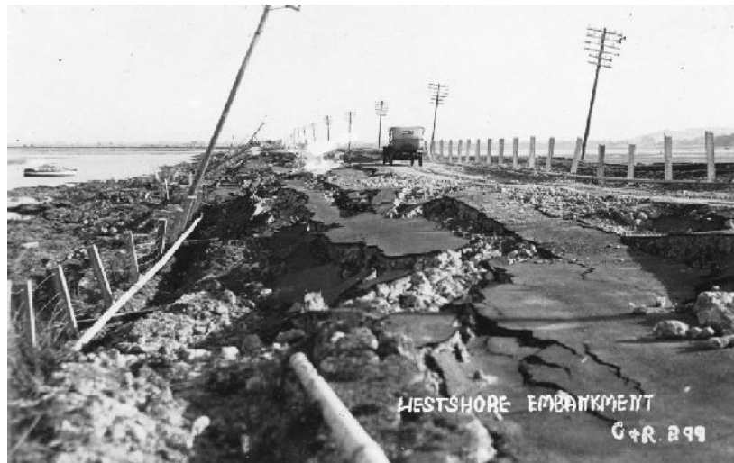
Figure B.2: Severe liquefaction and lateral spreading of the Westshore embankment ( from the archives of the MTG Hawke's Bay Museum )
