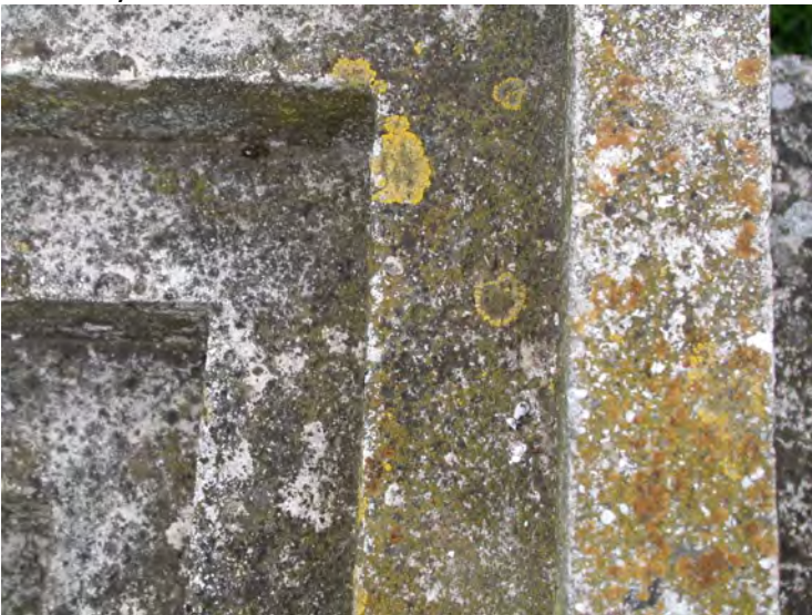
Fig. 6.34 Concrete with lichens Photo by Author
