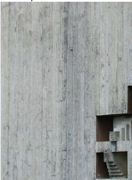
Fig. 5.15 Chapel Altar corner Vertical concrete formwork detail Photo by Author
