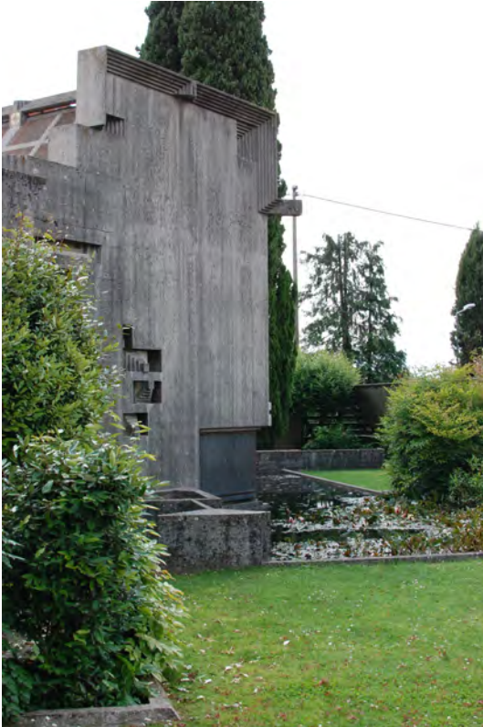
Fig. 5.14 Chapel northeast façade photo Photo by Author
