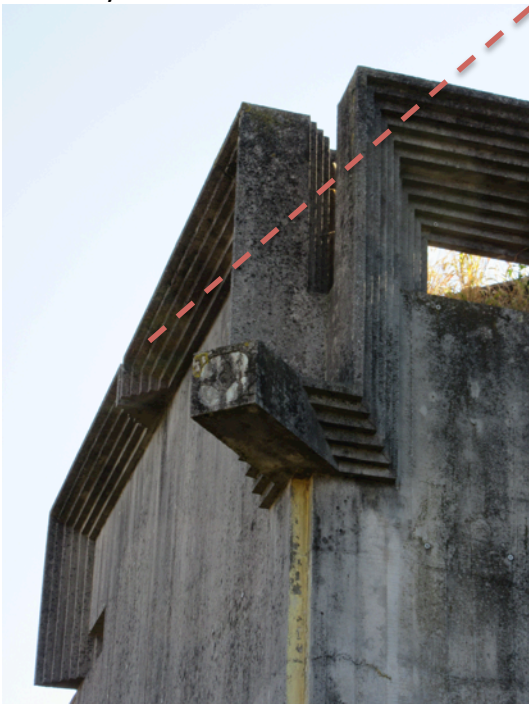
Fig. 3.8 Desired path of light (dash line) crossing through square opening in concrete wall Photo by Paul Emmons
