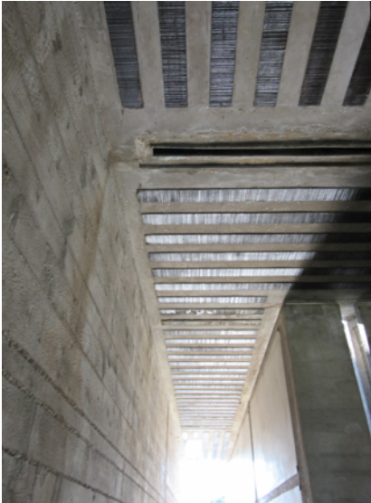
Fig.7.25 Corridoio ceiling Photo by Paul Emmons
