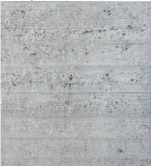
Fig. 6.32 Wood texture imprinted in concrete Photo by Author
