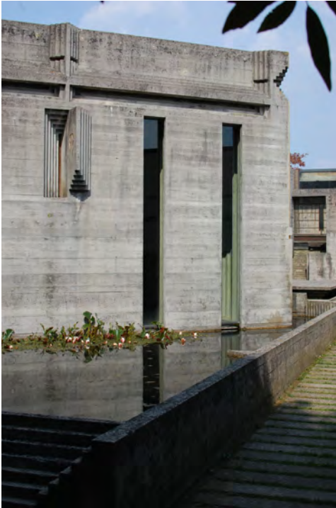
Fig. 6.31 Chapel southwest facade Photo by Author
