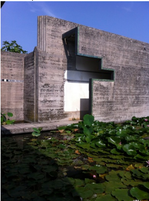
Fig. 7.41 End of corridoio area / path to padiglione Photo by author
