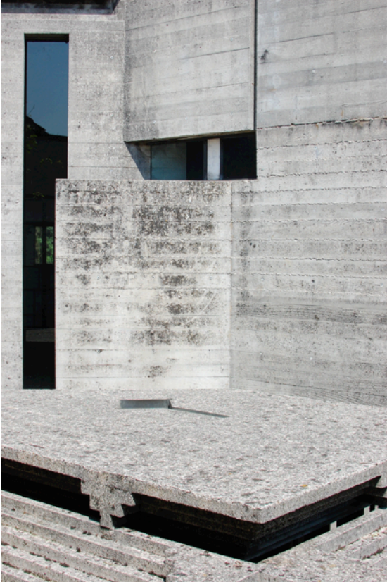
Fig. 3.3 Concrete slab lid Brion cemetery Photo by Author
