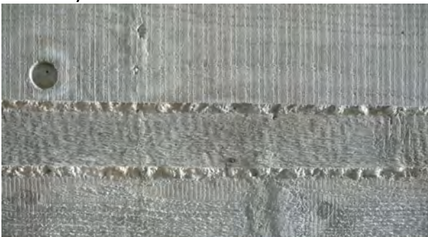
Fig. 6.27 Hammered concrete detail at corridoio Photo by Author
