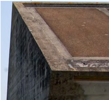
Fig. 6.9 Family pavilion roof material Photo by Author
