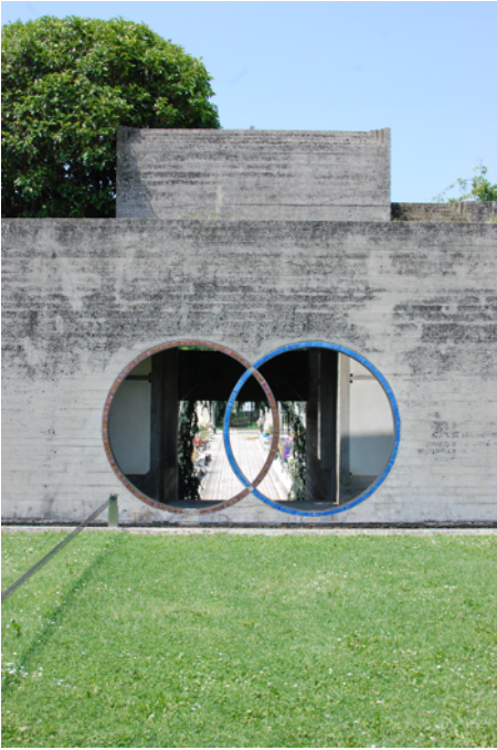
Fig. 7.34 Vesica Piscis opening on corridoio wall (exterior) Photo by author
