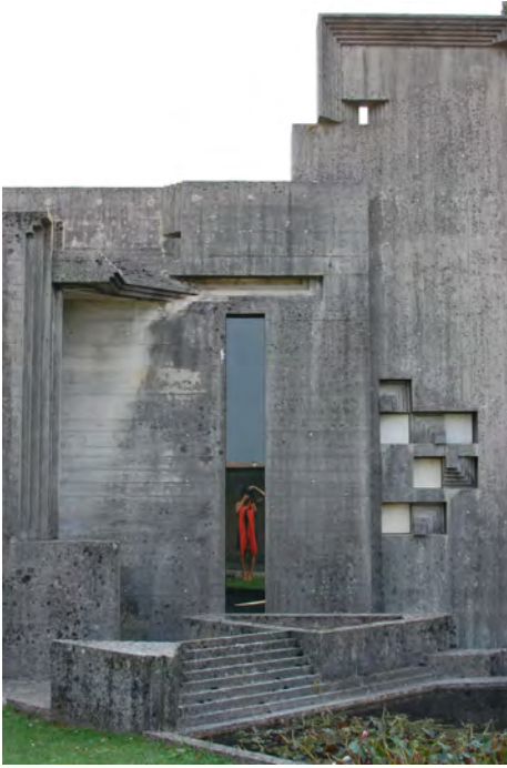
Fig. 6.35 Chapel northeast side façade Photo by Author
