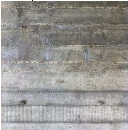
Fig. 6.26 Hammered concrete detail at corridoio Photo by Author
