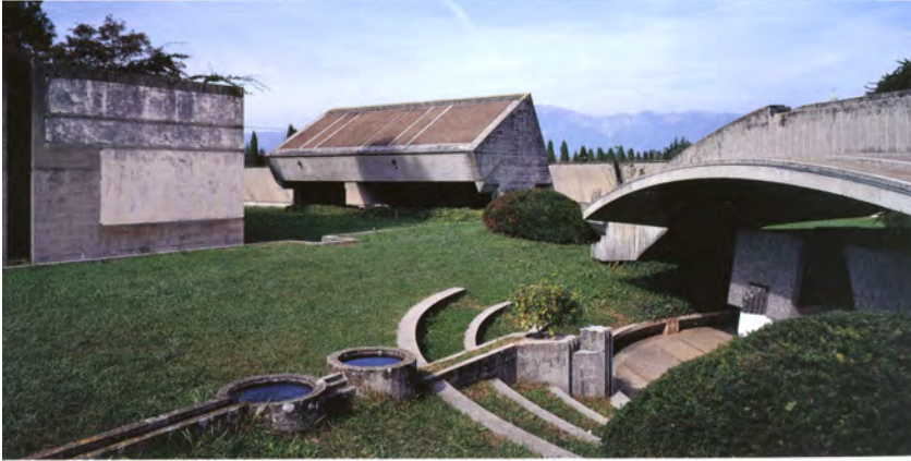
Fig. 6.1 Family pavilion (on the back) © Photo by Guido Pietropoli
