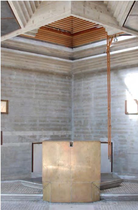
Fig. 5.16 Chapel Altar corner Interior horizontal formwork Photo by Author
