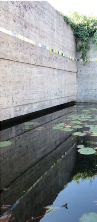
Fig. 9.6 'Floating' concrete wall, held by perimeter wall behind Photo by Paul Emmons
