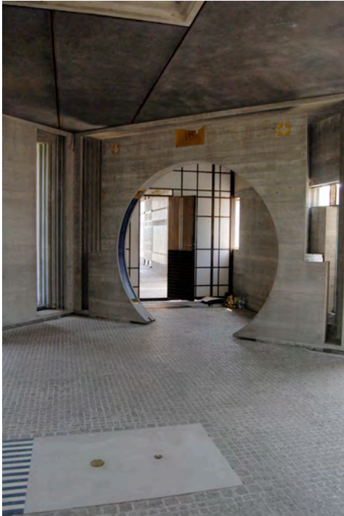
Fig. 8.13 "Moon" concrete opening at chapel Photo by Author
