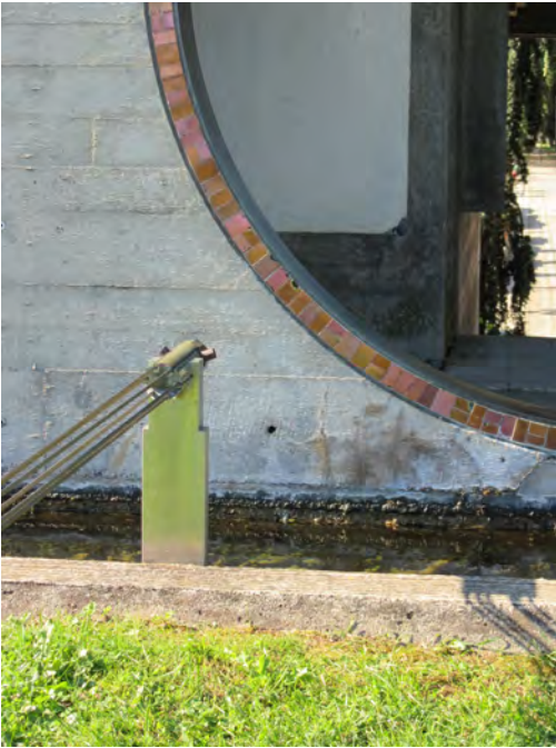
Fig. 8.29 Cable structure with spring Photos by Paul Emmons
