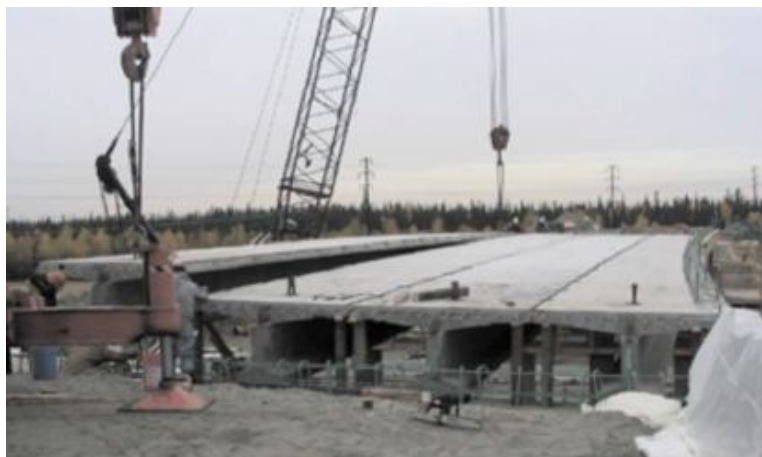
Figure 5 DBT bridge system. Obtained from (Li et al. 2010)
