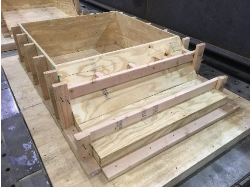
Figure 27 Inverted T-beam formwork (left). Inverted T-beam C.I.P. Topping formwork (right)
