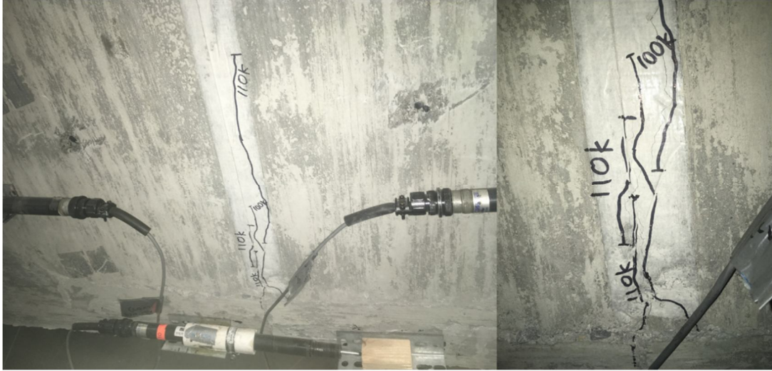
Figure 84 Welded connection failure test - C.I.P. cracking at 110 kips
