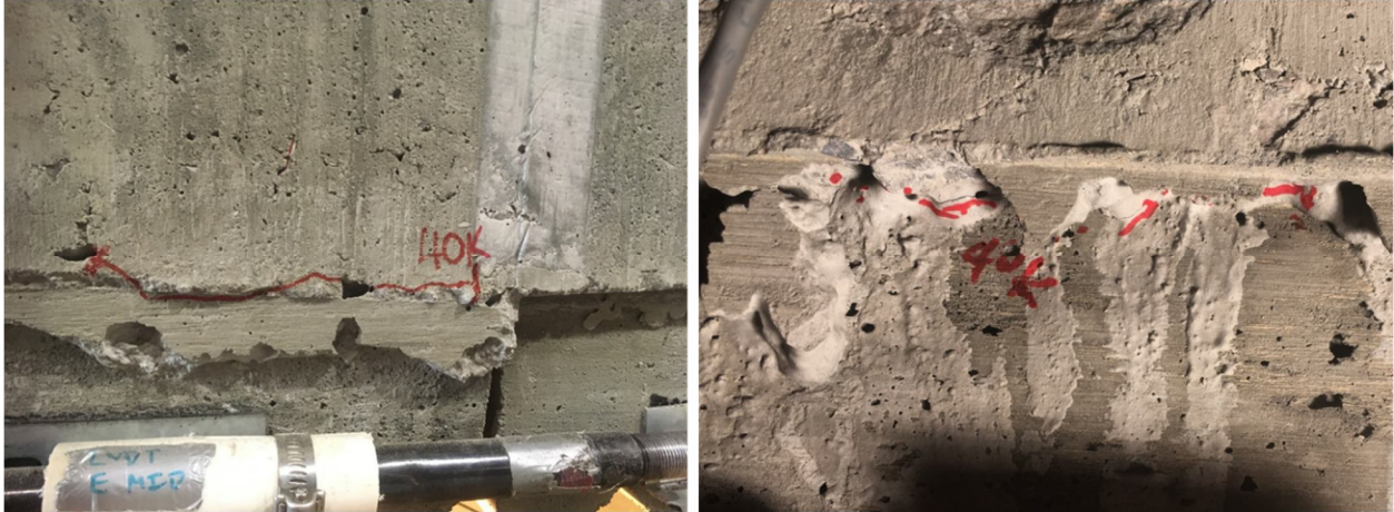
Figure 65 Monotonic load test to failure - cracking at 40 kips actuator load
