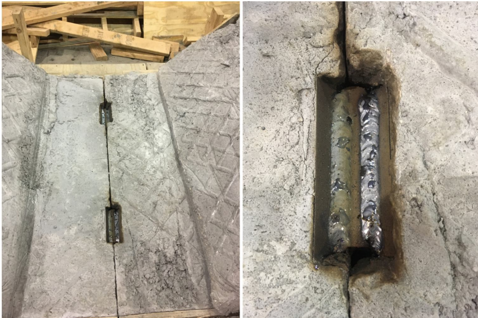
Figure 32 Welded connection after welding completed
