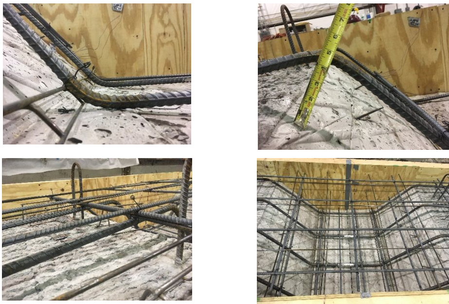
Figure 34 Challenges with reinforcement placement. (Top-left) Inadequate cover at the tapered web-flange interface. (Top-right) Too much cover at extended web-tapered web region. (Bottom-left) Bottom mat of reinforcement clashing with top mat. (Bottom-right) Reinforcement placement within joint region.
