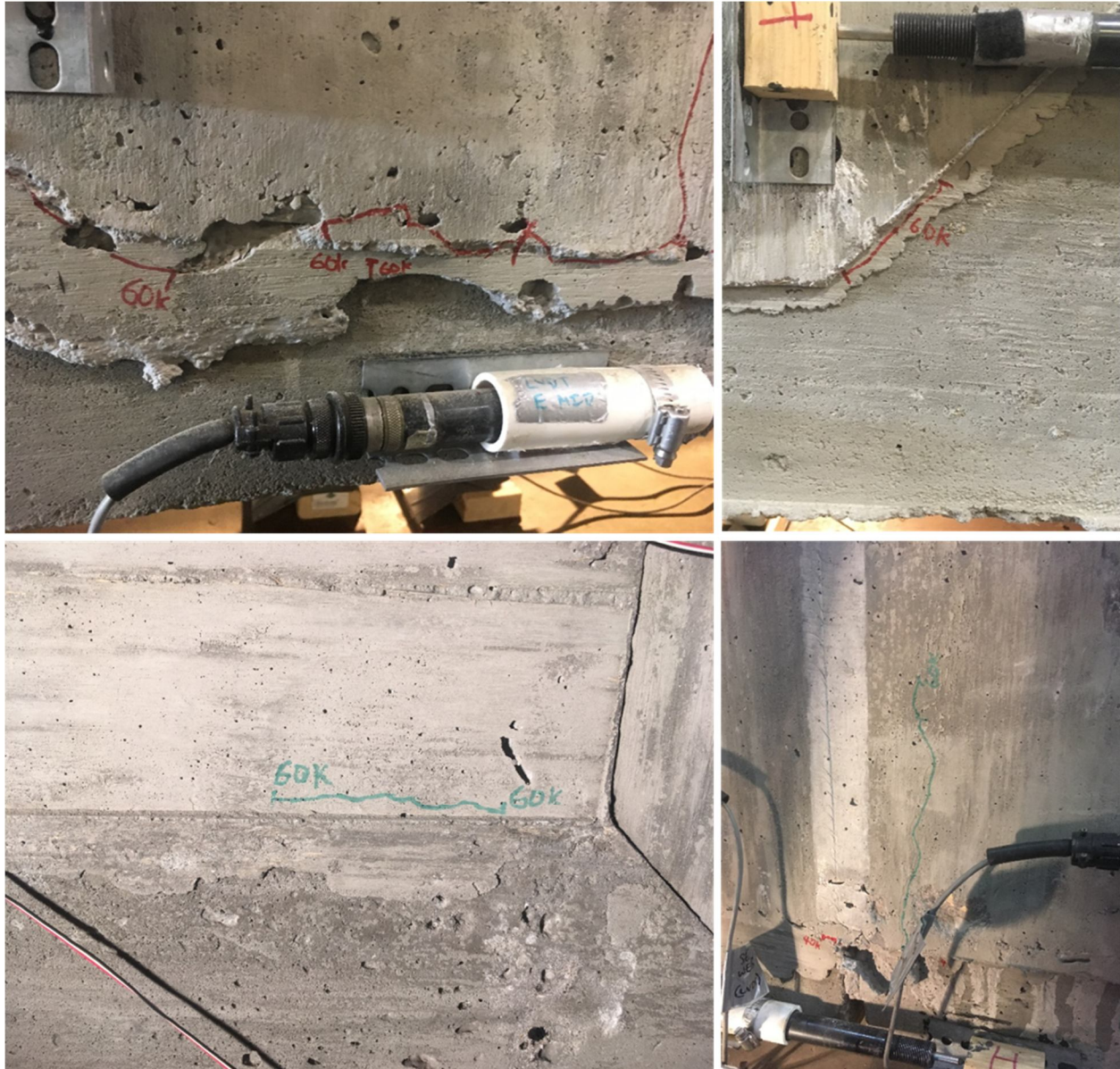
Figure 67 Monotonic load test to failure - cracking at 60 kip actuator load
