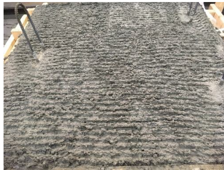
Figure 23 Raked surface finish above extended web region
