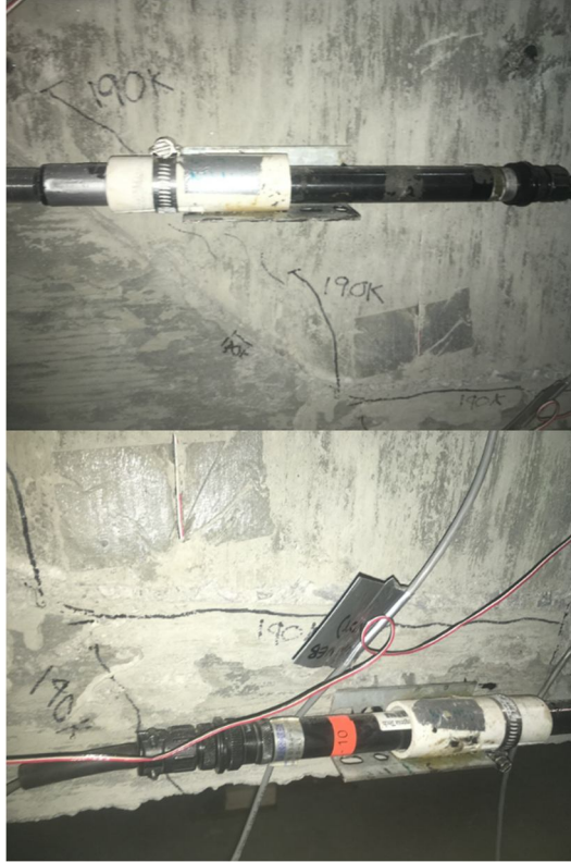
Figure 86 Welded connection failure test - interface cracking at 190 kips
