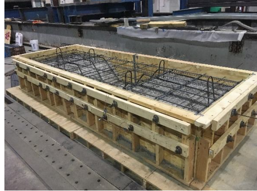
Figure 27 Inverted T-beam formwork (left). Inverted T-beam C.I.P. Topping formwork (right)
