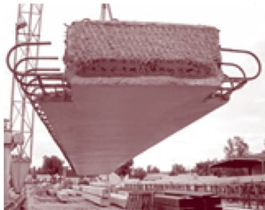
Figure 7 Poutre Dalle beam unit. Obtained from (Mary Lou Ralls et al. 2005)
