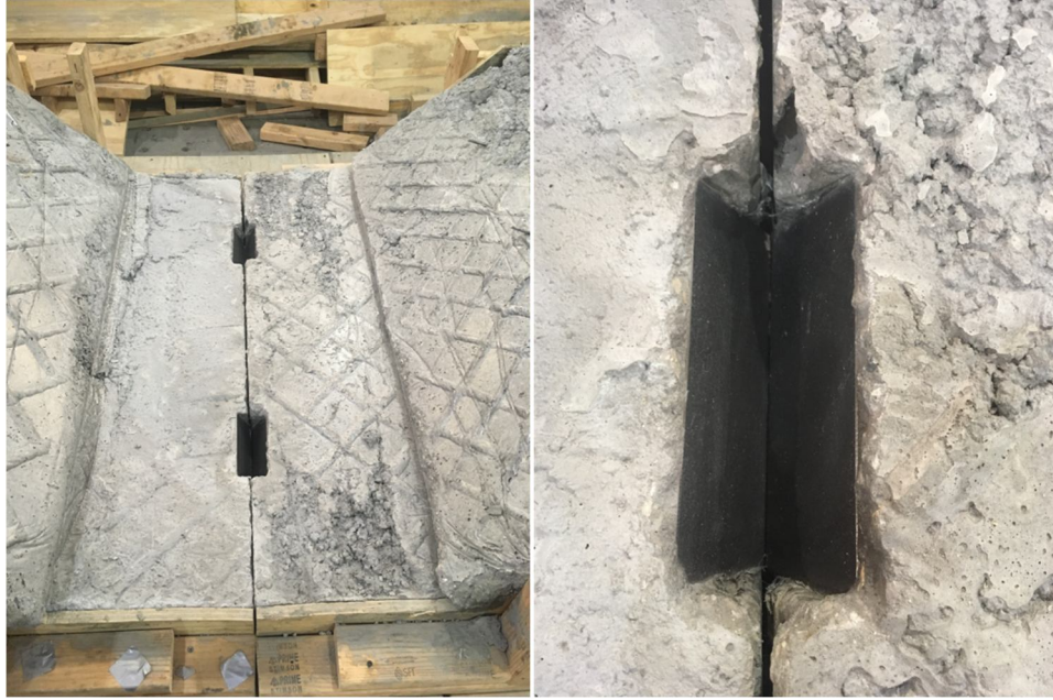
Figure 31 Embedded plate connection prior to welding
