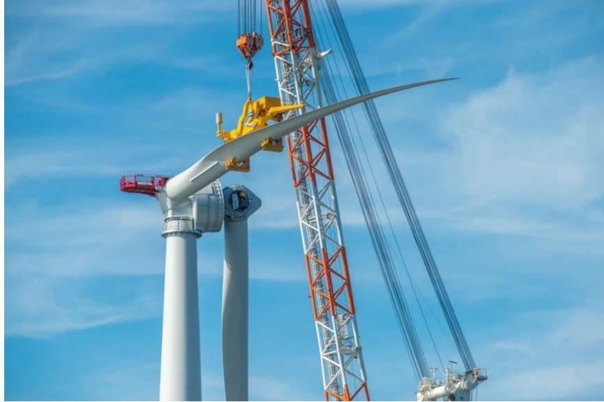
Figure 2: The GE Wind Turbine in the Block Island wind farm project [6].
