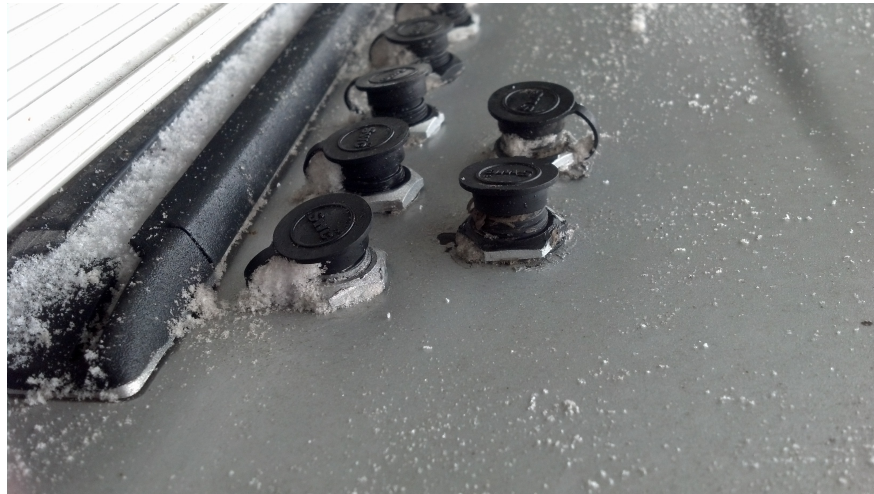
Figure 3.28: Example of roof top penetrations.
