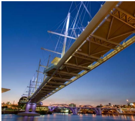
Figure 8 The Kurilpa Bridge, in Brisbane, Australia is the world’s largest [50]
