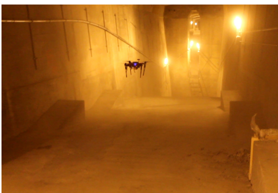
(b) Flight inside VTTI's smart bridge
