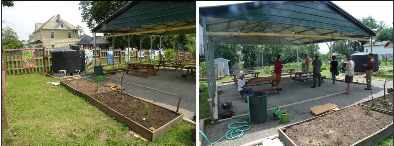
Fig. 9 Rainwater harvesting systems at Hurt Park Community Garden, photo on left shows a 1500 gallon ( 5.7 \text{ m}^3 ) barrel to the left of the pavilion; photo on the right shows a second barrel to the right of the pavilion (photos: third author 2013)
