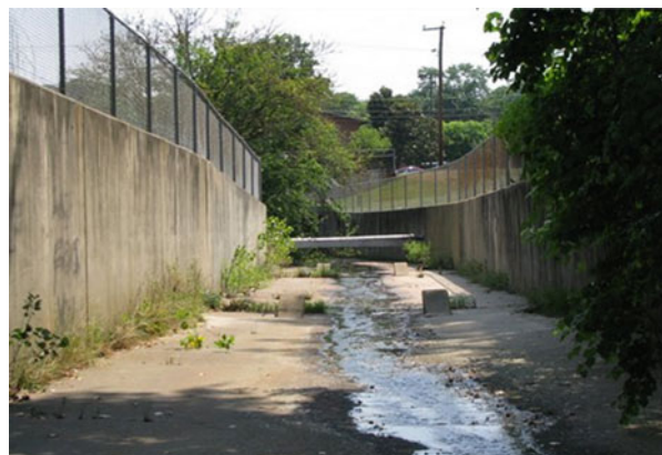
Fig. 7 Reedy Creek, Richmond, Virginia (USA). Impervious surfaces have replaced the natural stream channel and habitat. The channel was designed to remove stormwater from residential, commercial, and industrial land uses (Photo by the first author)
