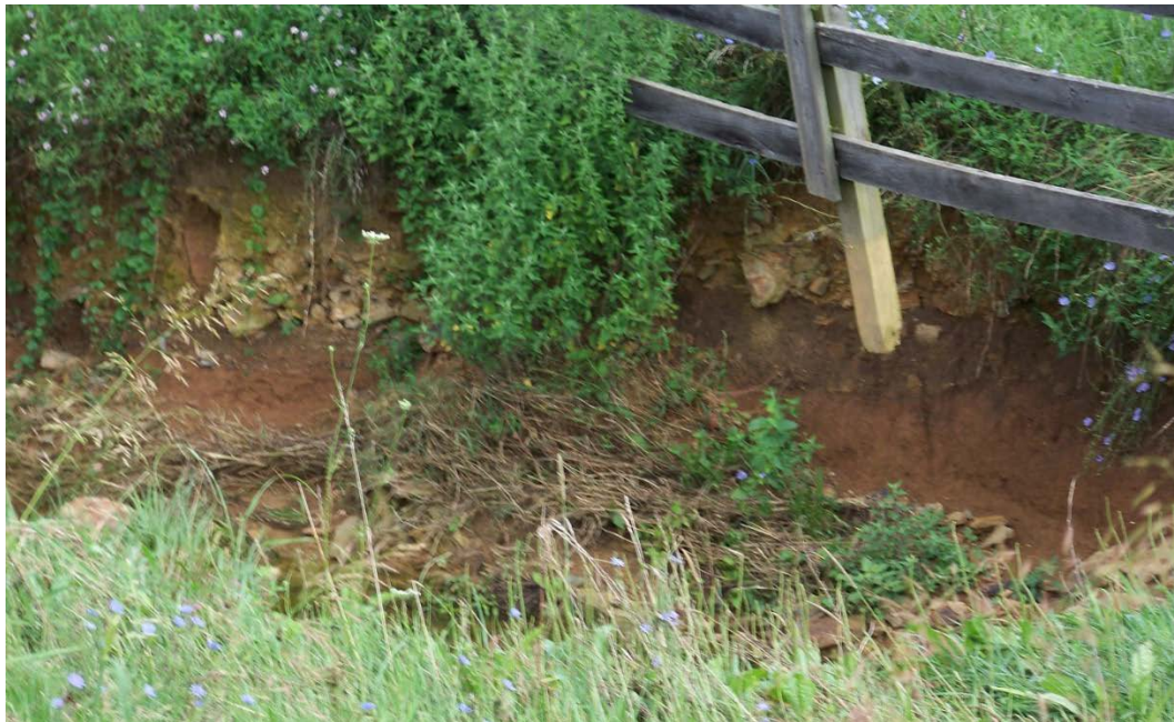
Fig. 14 Erosion on Heritage Point Urban Farm's property caused from unchanneled stormwater runoff from the industrial park's buildings and parking lots (photo - first author 2013)
