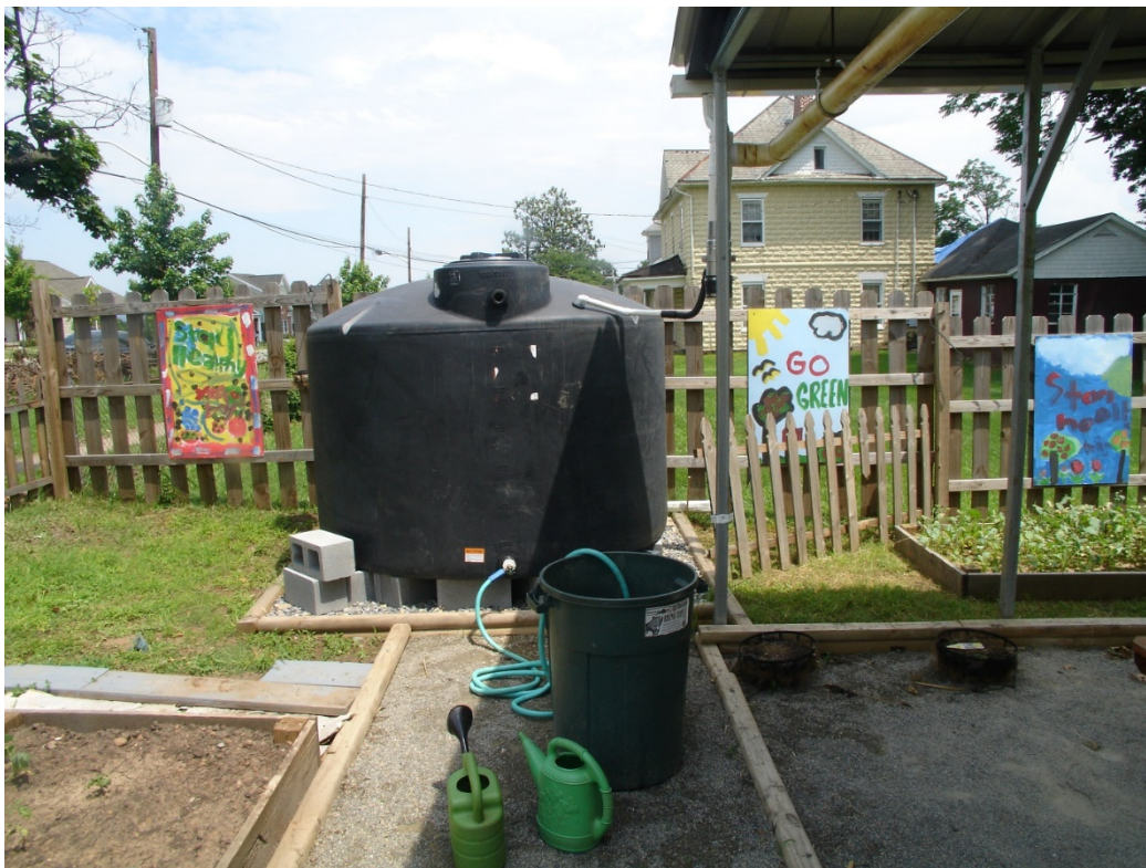
Figure 1.6 Rainwater harvesting system at Hurt Park Community Garden (Photo by James B. Campbell 2013)
