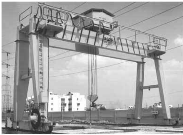
(a) Gantry crane.
