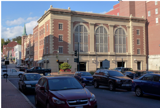
Staunton, Virginia parking garage 103
