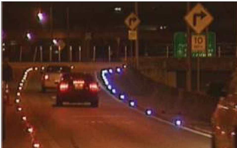
Figure 6. Photo. Horizontal curve IPM system with a reverse chase pattern (courtesy of Intelligent Traffic Equipment Marketing Ltd.).
