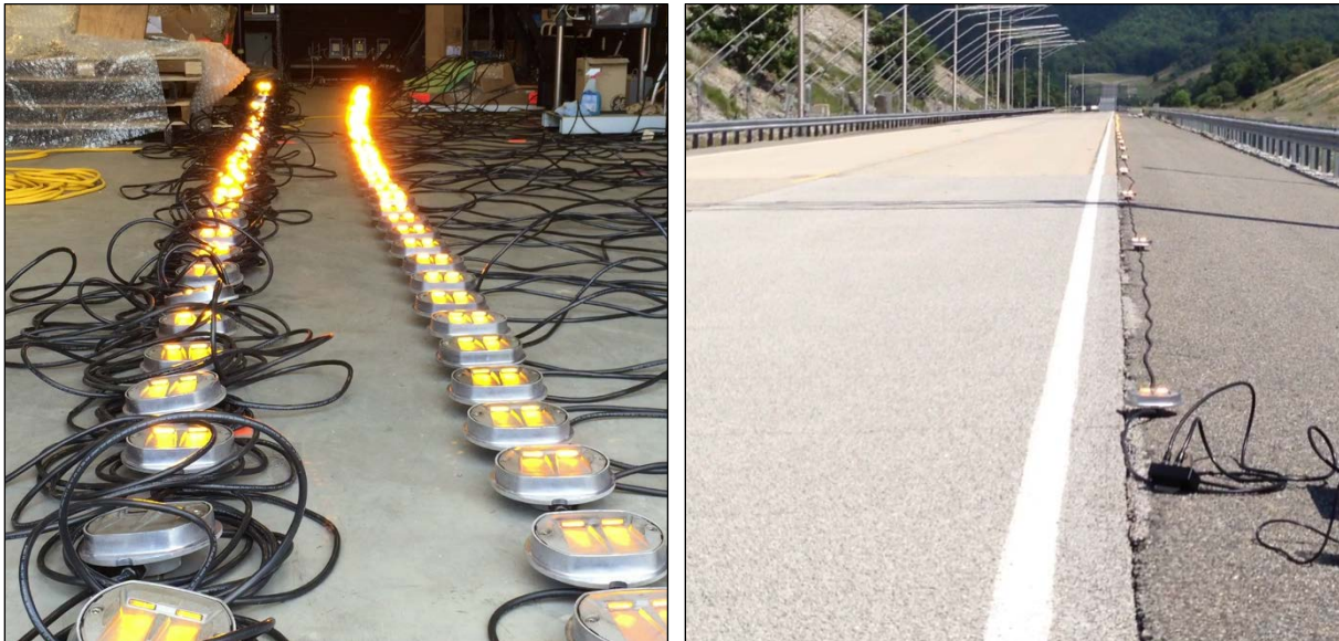
Figure 3. Photo. Temporary LaneLight™ delineation system.
