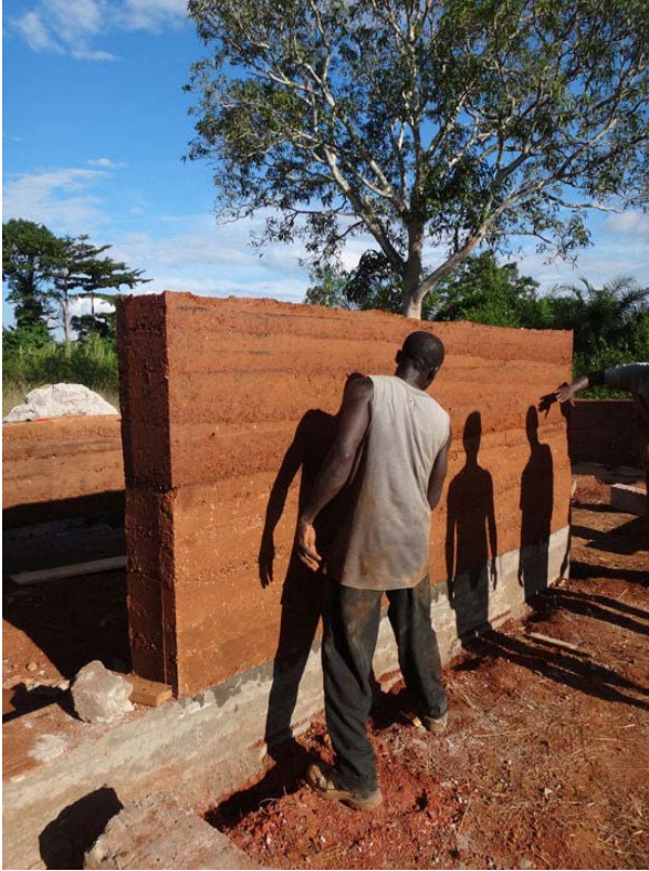
(8) Constructing compressed earth wall
