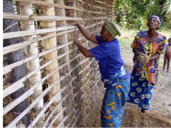
(7) Creating framing reinforcement for compressed earth
