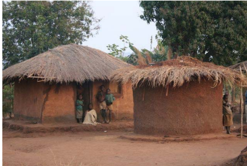
(3) Village Homes constructed of compressed earth
