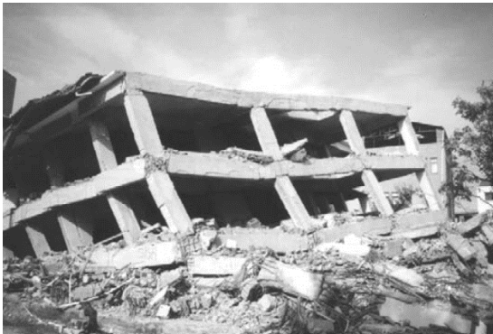
c) Collapsed building following Izmit, Turkey earthquake. Hassan (2011)
