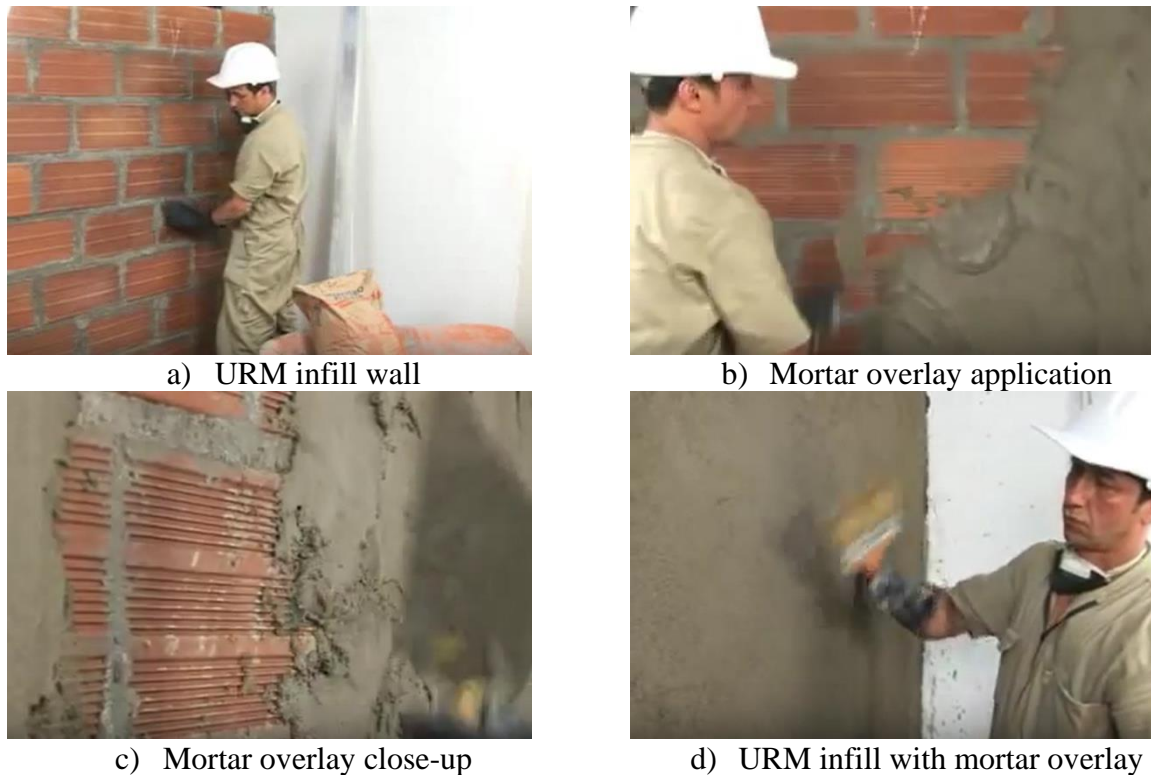
Figure 5-6. URM infill with mortar overlay construction sequence.
