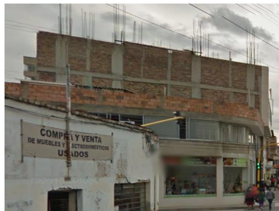
b) Side view of a RCF with URM infills
