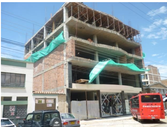
a) Typical RCF with URM infills.
