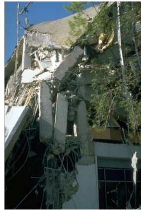
a) Structure collapse Kaiser Permanente Building, Northridge earthquake. (photo credit, G. Edstrom)
