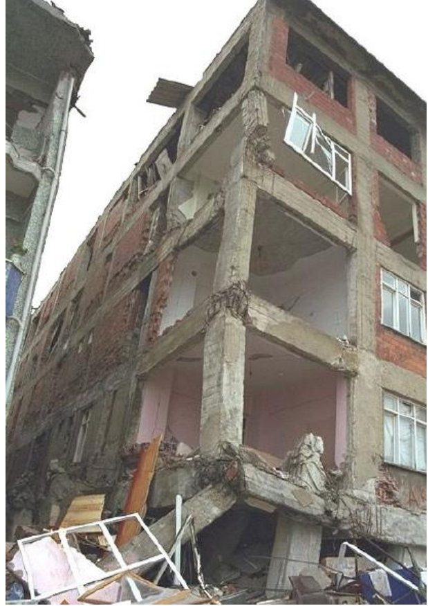
b) Partial Building Collapse due to failure of beam-column joints in the Izmit, Turkey earthquake. (photo credit, NISEE)
