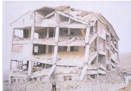
d) Joint failure and partial building collapse Erzincan, Turkey earthquake. Hassan (2011)
