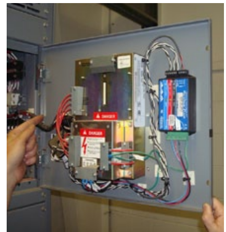
Installed Energy Management System
