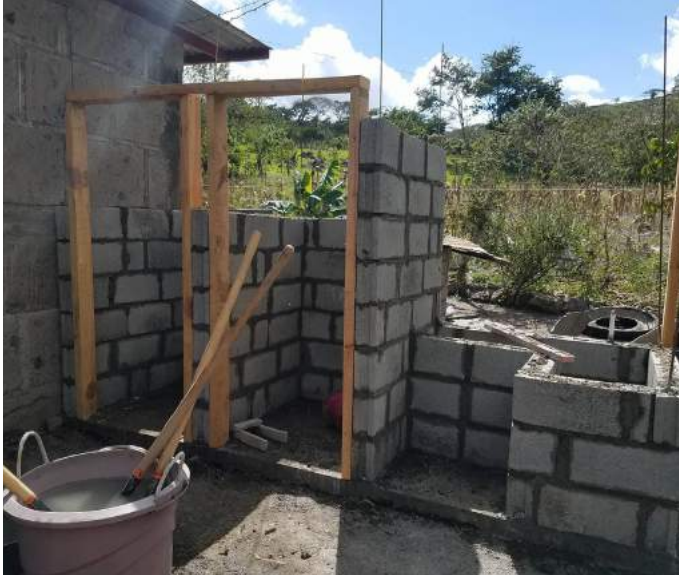
Concrete scaffolding for a sanitation project. The use of concrete versus other materials allowed for a higher level of sanitation. (Credit: L. Davies)
