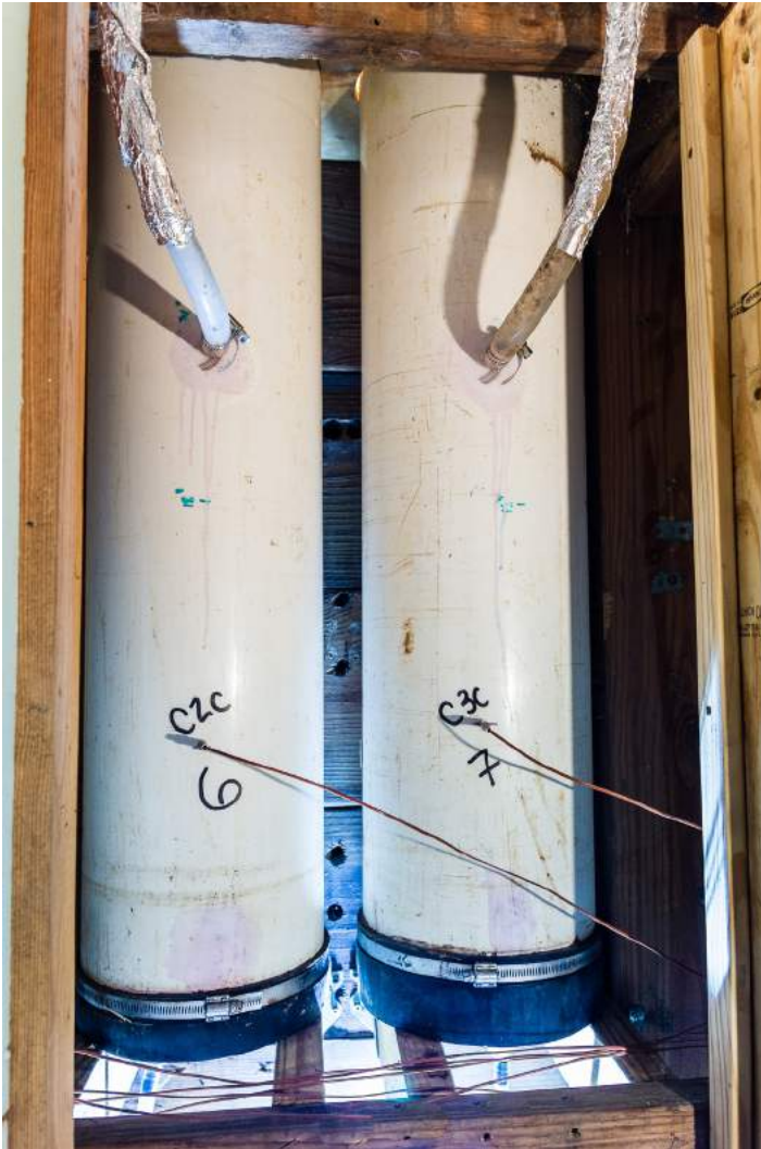
“Mini septic fields” are set up inside the soil bunker in which water enters through the top and discharges out the bottom. It takes the water two to three days to completely flow through, depending on the characteristics of the soil inside. The discharged water is tested for E. coli using source tracking.
