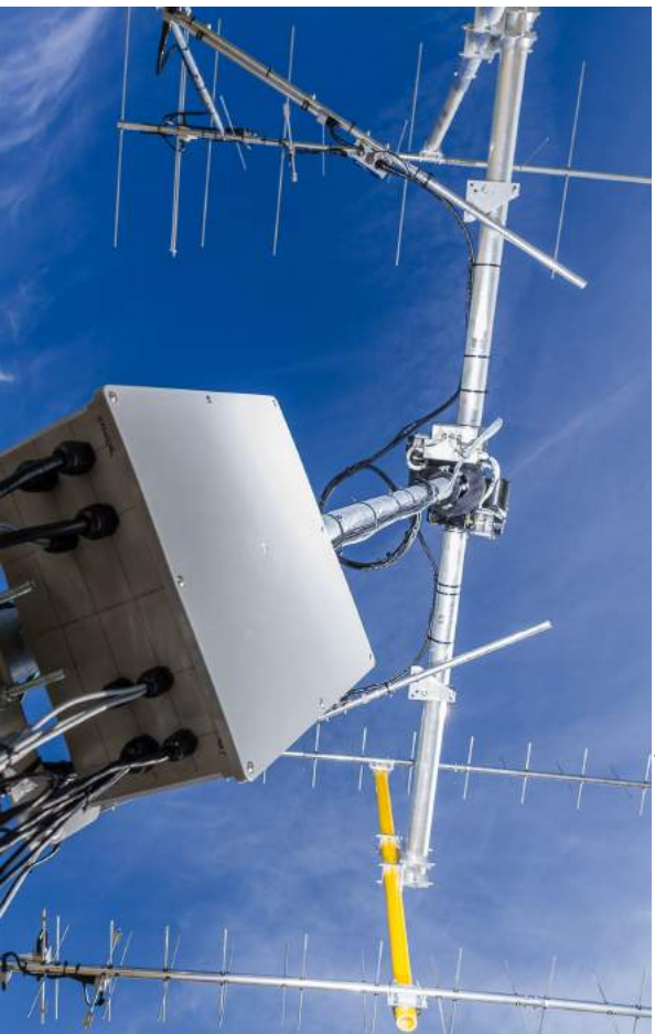
A view of the VHF/UHF subsystem currently in place at the Ground Station. It is primarily used to communicate with spacecraft such as CubeSats and SmallSats to download mission data.
